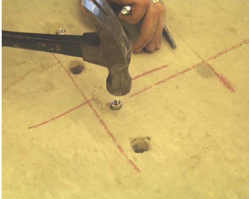
Figure 109. Photo. Concrete anchor installation step 6.
