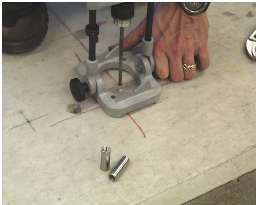
Figure 108. Photo. Concrete anchor installation step 3.
