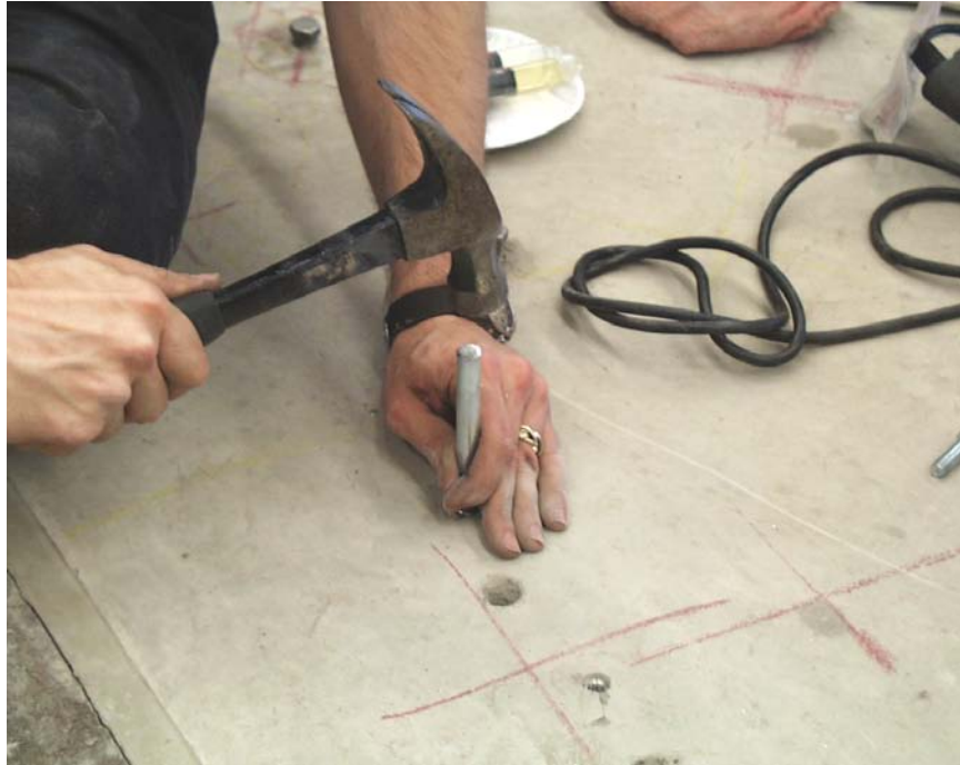
Figure 110. Photo. Concrete anchor installation step 7.
