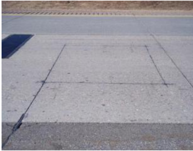
Photo 7 – Trailing Loop Sensor
