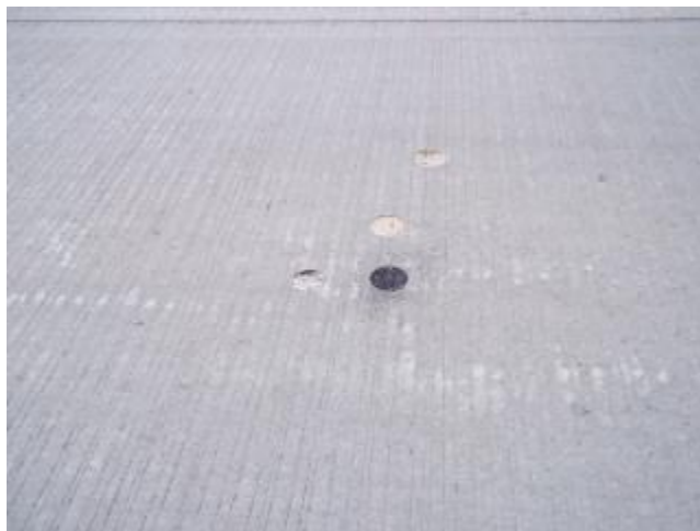
Figure 4-1 – Core Sample Patches at 220 Feet Prior to WIM
