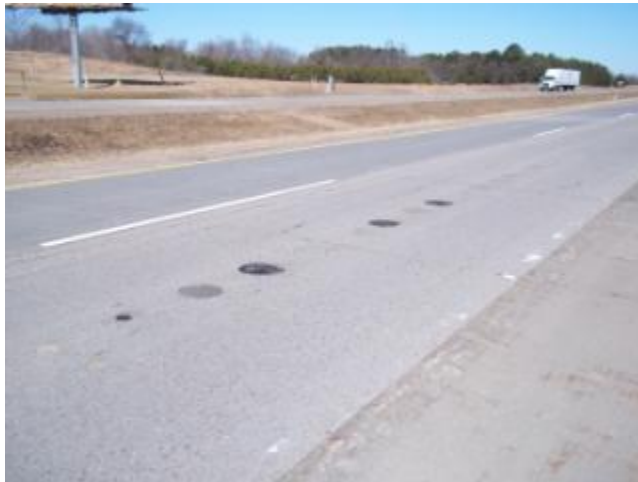
Figure 4-2 – Core Sample Patches at 680 Feet Prior to WIM
