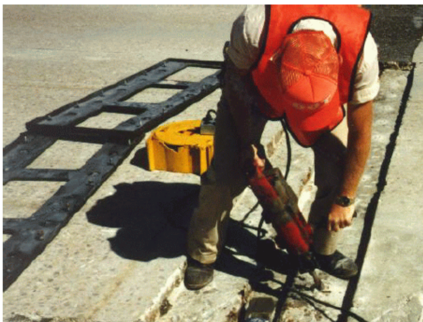
Figure 10 - Drilling Frame Anchor Holes 123-429-900-970.jpg
