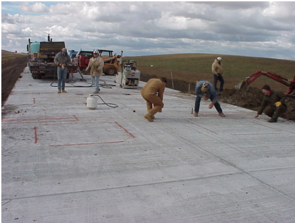
Figure 4 - Laying out Site
