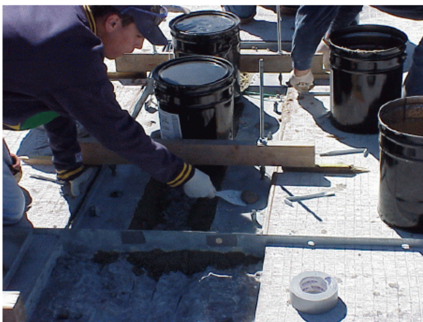
Figure 15 - Removing Excess Epoxy 123-429-901-000.jpg
