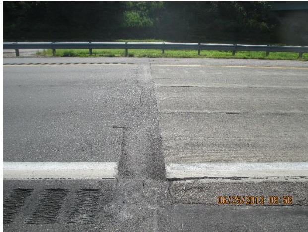
Photo 3-1 - Pavement Transition 12 Feet Prior to WIM Scales
