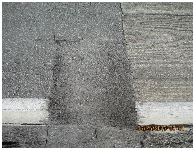
Photo 3-2 – Pavement Transition 12 Feet Prior to WIM Scales (2)
