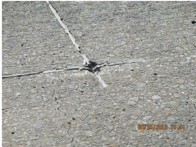
Photo 4-2 – Missing Loop Sealant – Trailing Loop Sensor
