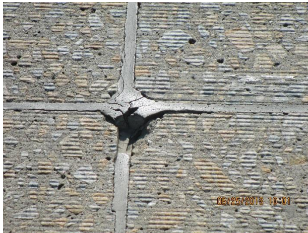
Photo 4-1 – Missing Loop Sealant – Leading Loop Sensor
