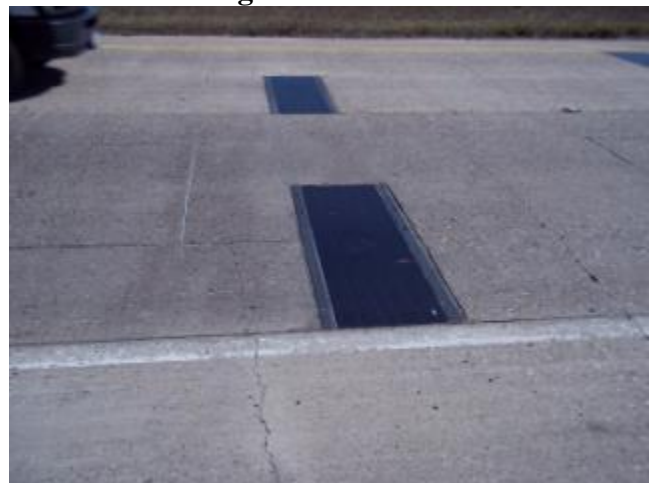
Photo 6 – Trailing WIM Sensor
