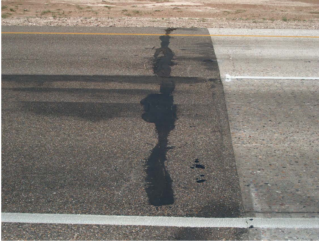
Figure 4-2 Photo of the AC/PCC Pavement interface – 480100 - 27-Apr-2005
