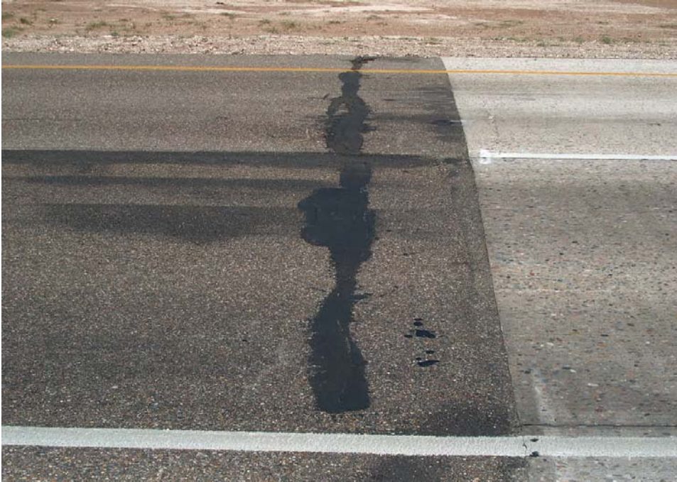
Photo 6-15 - TO_9_48_2.48_100_Transverse_Crack.JPG
