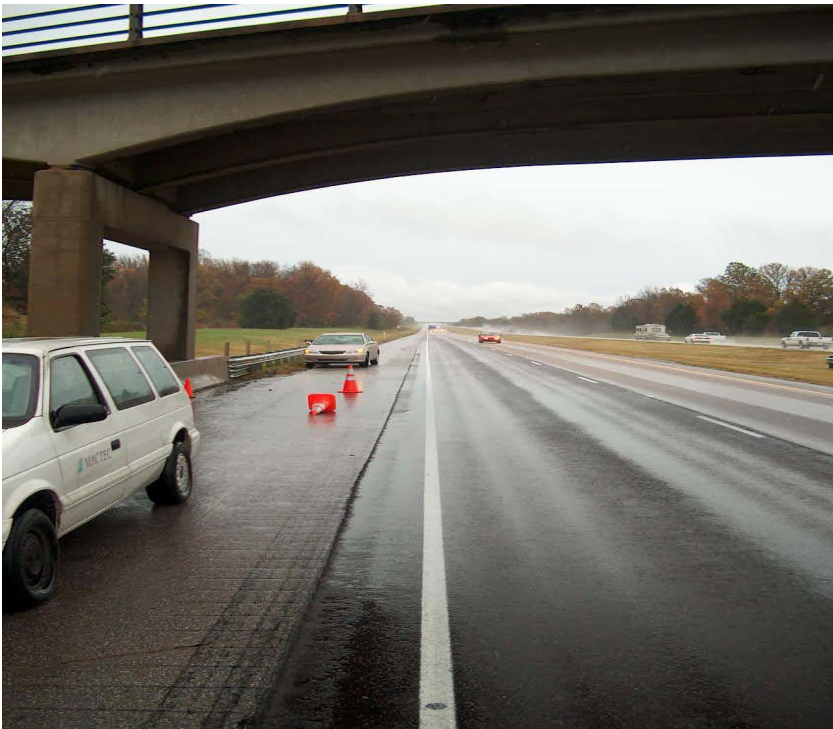
Figure 13-2 Pavement Condition at Site 470600 (Upstream)
