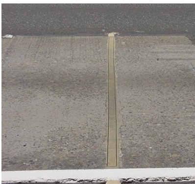
Figure 28 - Piezo Class II sensor
