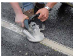
Diamond grinder (rough grinding) Belt sander (finishing)
