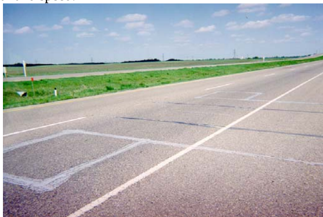
Figure 27 - Loop sensors
