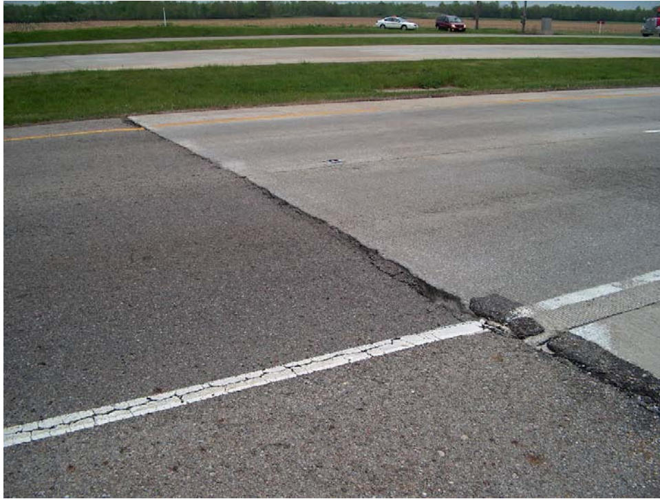
Figure 4-1 - Photo of the Asphalt to PCC transition - 390100 - 12-May-2005
