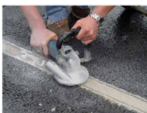
Diamond grinder (rough grinding) Belt sander (finishing)
