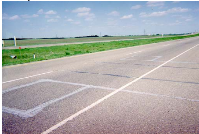
Figure 27 - Loop sensors
