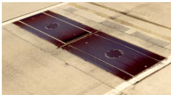
Figure 24 – Single Load Cell scales
