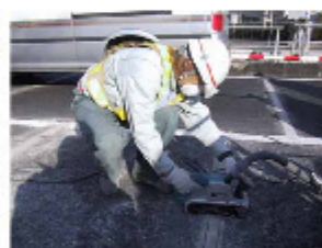
Diamond grinder (rough grinding) Belt sander (finishing)
