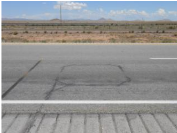
Photo 7 – Trailing Loop Sensor
