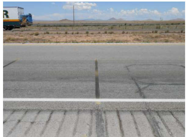
Photo 6 – Trailing WIM Sensor
