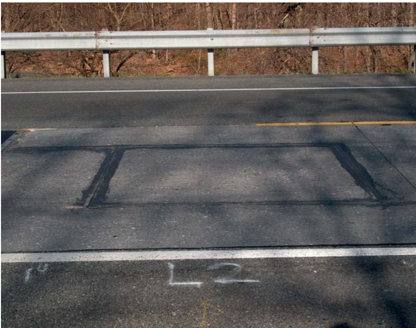
Photo 8 – Trailing_Loop_Sensor_TO_11_24_2.55_0500_03_21_06.jpg
