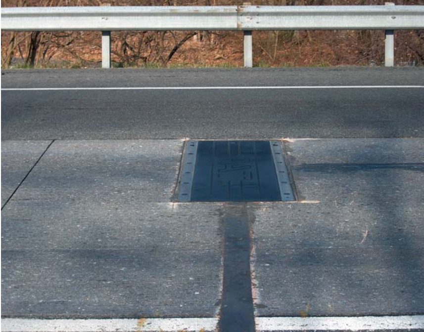
Photo 7 – Trailing_Weight_Sensor_TO_11_24_2.55_0500_03_21_06.jpg
