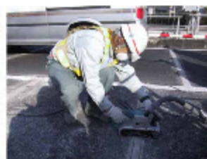
Diamond grinder (rough grinding) Belt sander (finishing)
