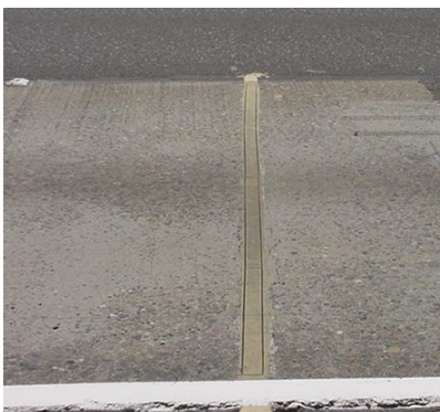
Figure 28 - Piezo Class II sensor
