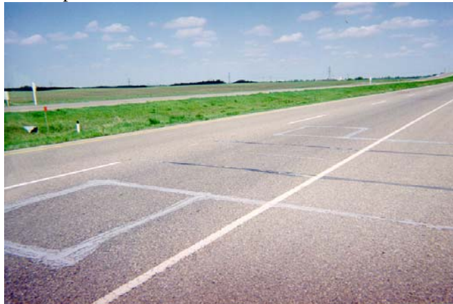
Figure 27 - Loop sensors
