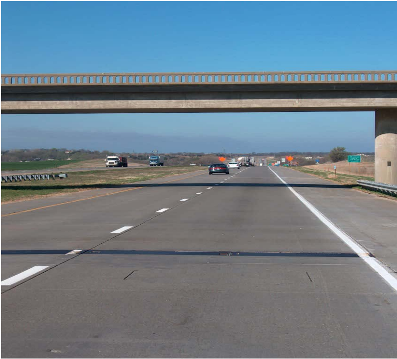
Figure 13-1 Pavement Condition in Downstream Direction at 200200
