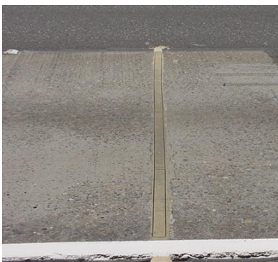
Figure 28 - Piezo Class II sensor
