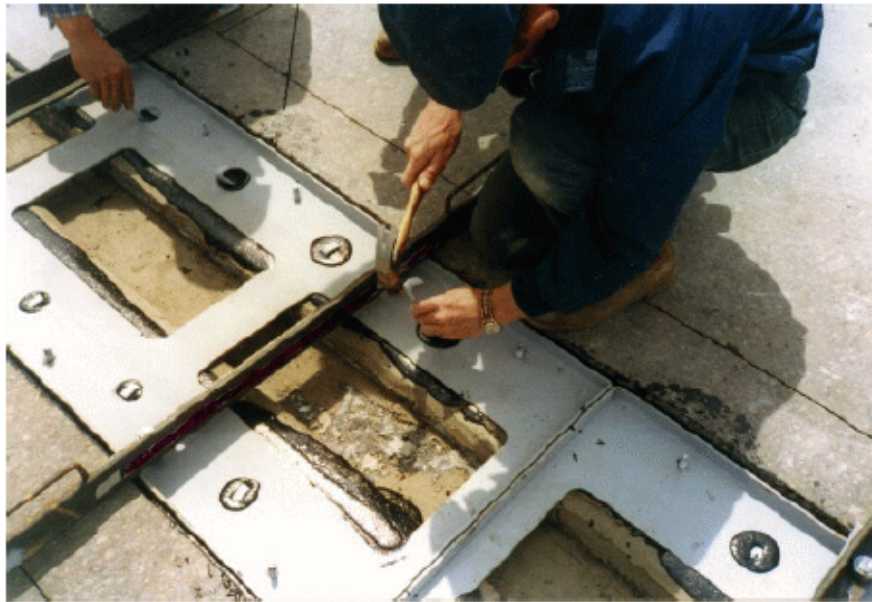
Figure 16 - Driving in Anchors
