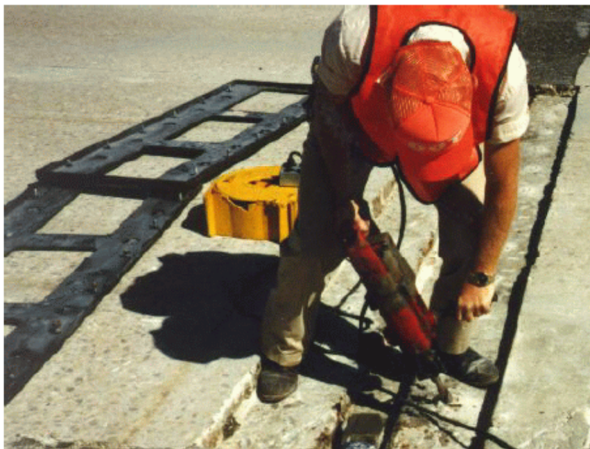
Figure 10 - Drilling Frame Anchor Holes 123-429-900-970.jpg
