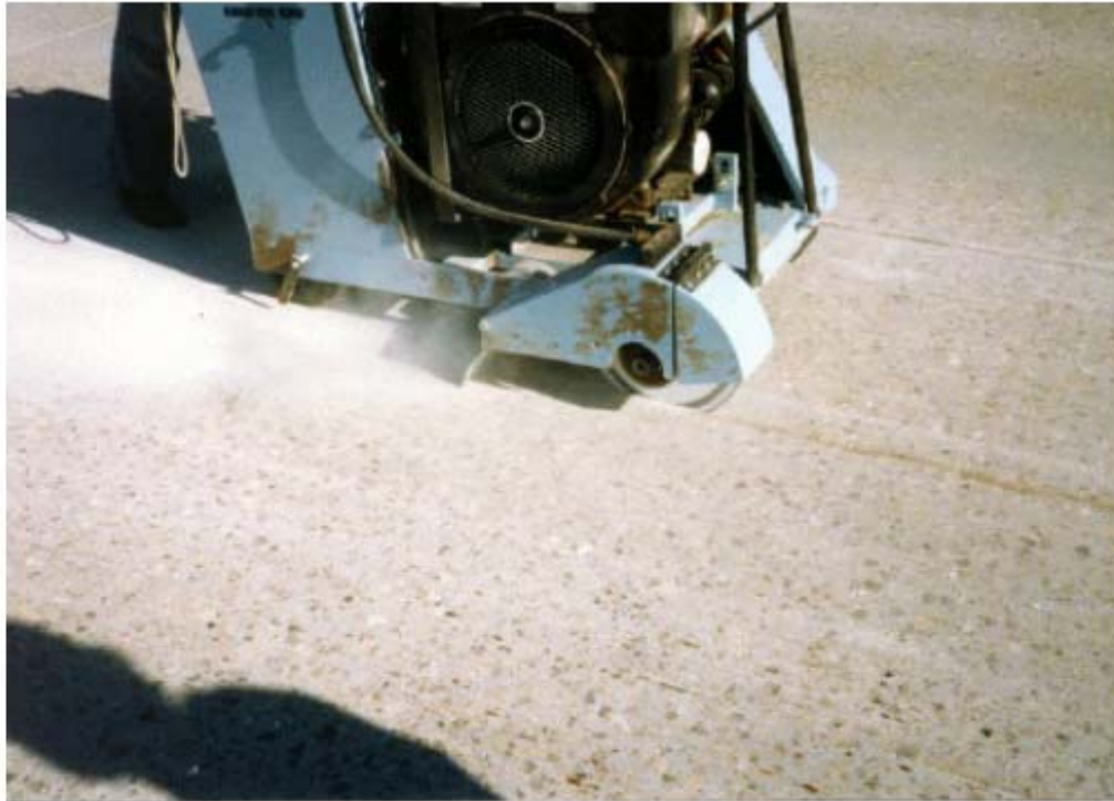
Figure 6 - Cutting Frame Recess
