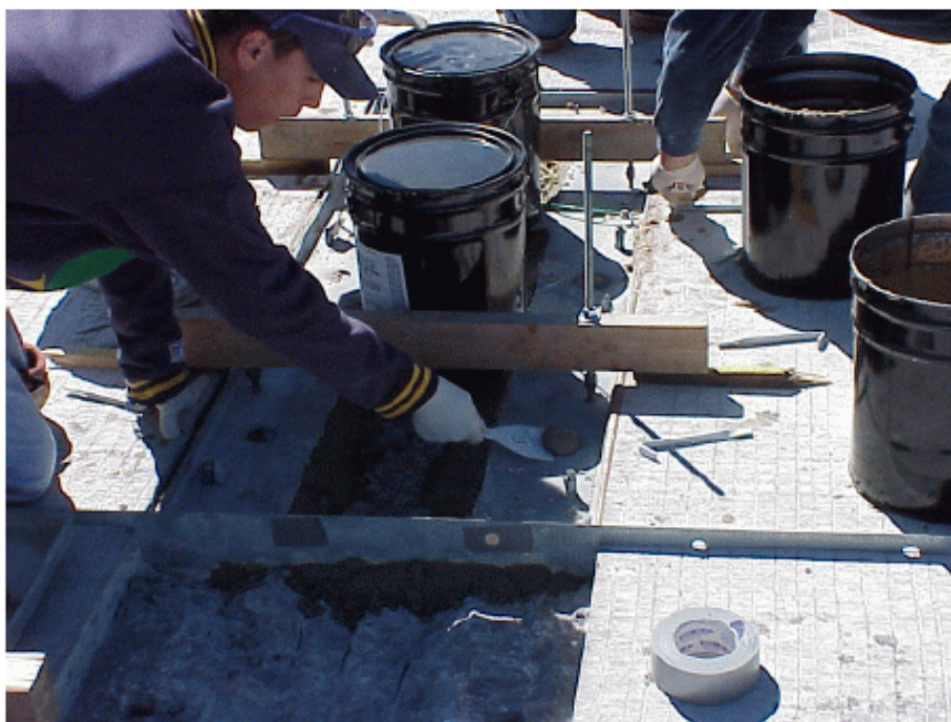
Figure 15 - Removing Excess Epoxy 123-429-901-000.jpg
