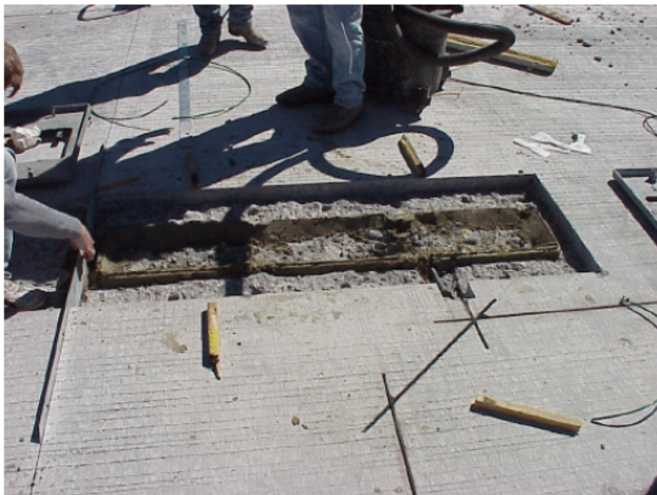
Figure 13 - Creating Cement Walls
