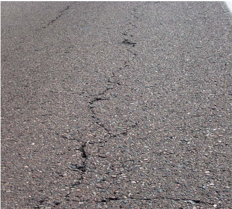
Figure 13-2 Alligator Cracking of Asphalt Pavement at 060500
