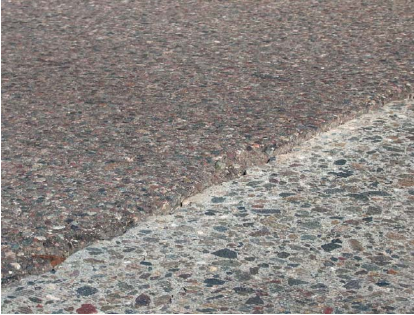
Figure 13-5 Faulting at Asphalt to PCC Pavement Transition at 060500
