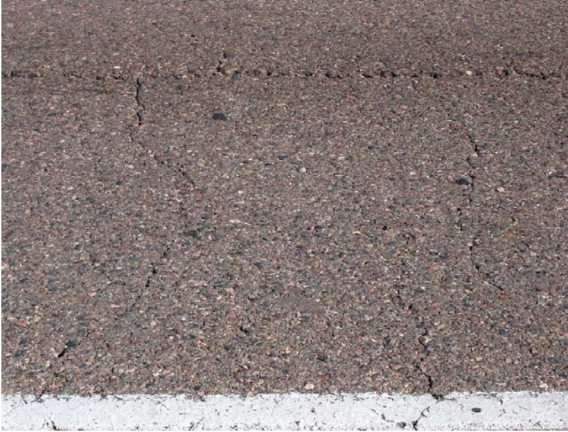
Figure 13-3 Block Cracking of Asphalt Pavement at 060500
