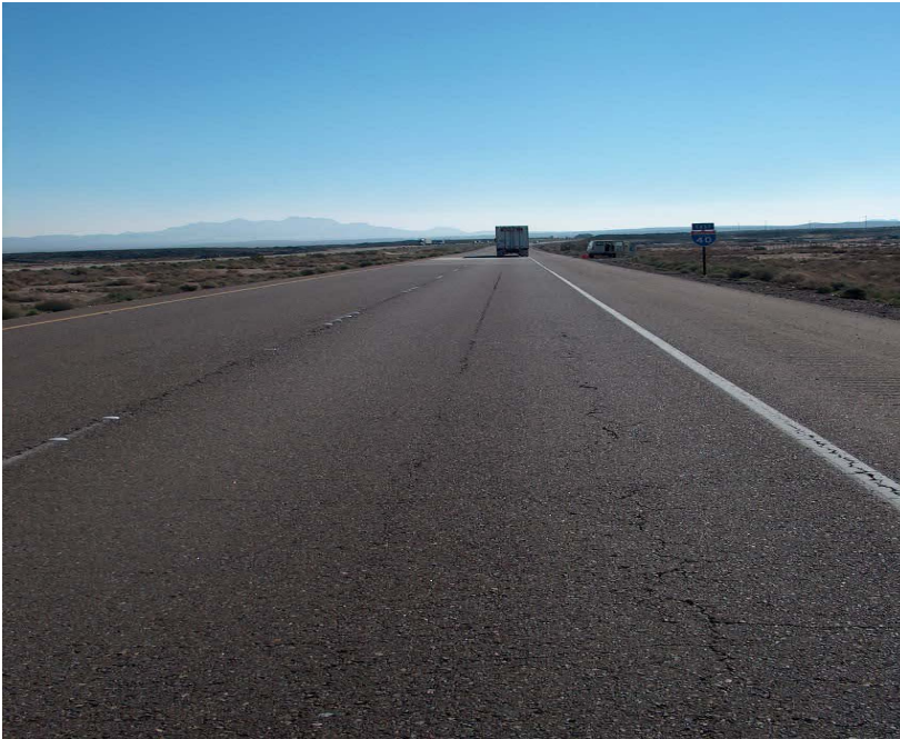
Figure 13-1 Longitudinal Cracking at 060500
