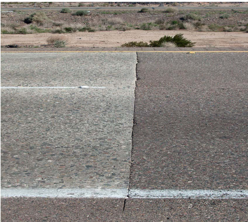
Figure 13-6 Faulting at PCC to Asphalt Pavement Transition at 060500
