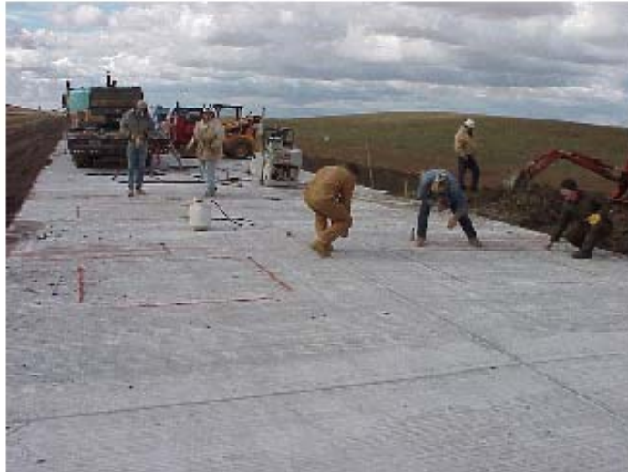
Figure 4 - Laying out Site
