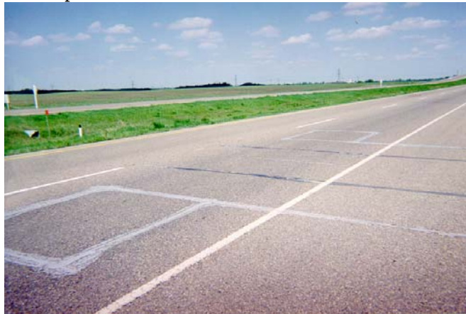
Figure 27 - Loop sensors
