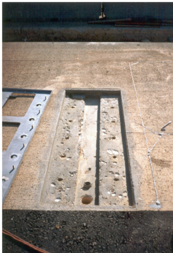
Figure 7 - Excavated Recess
