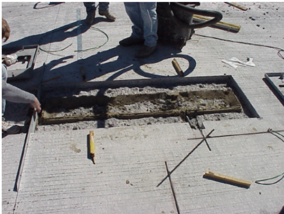
Figure 13 - Creating Cement Walls
