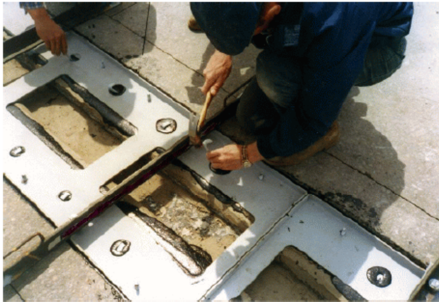
Figure 16 - Driving in Anchors
