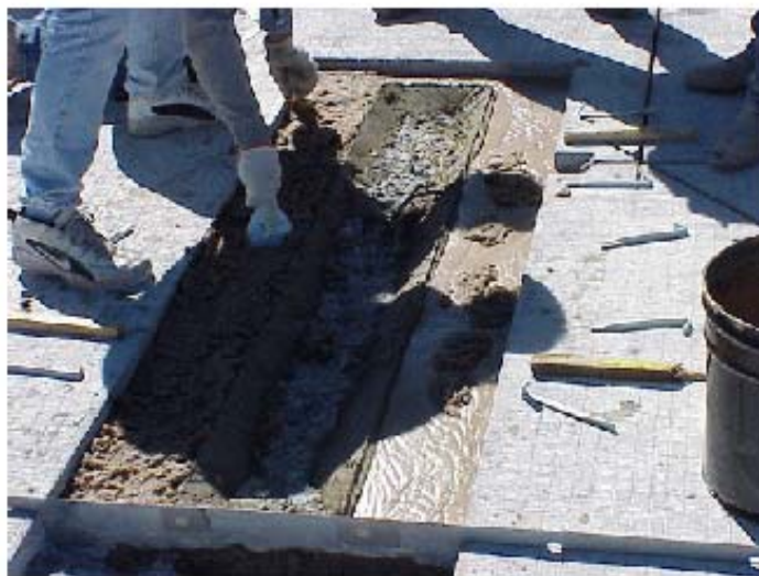
Figure 14 - Pouring Epoxy
