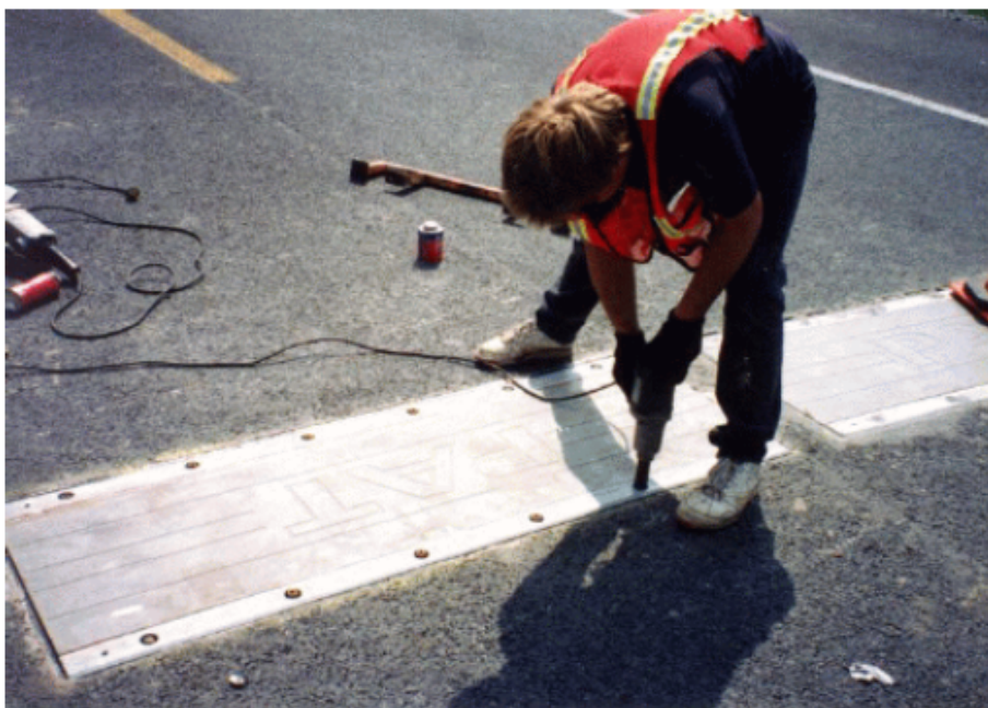
Figure 21 - Tightening Securing Rails
