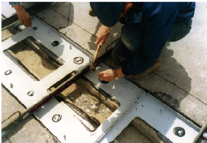
Figure 16 - Driving in Anchors
