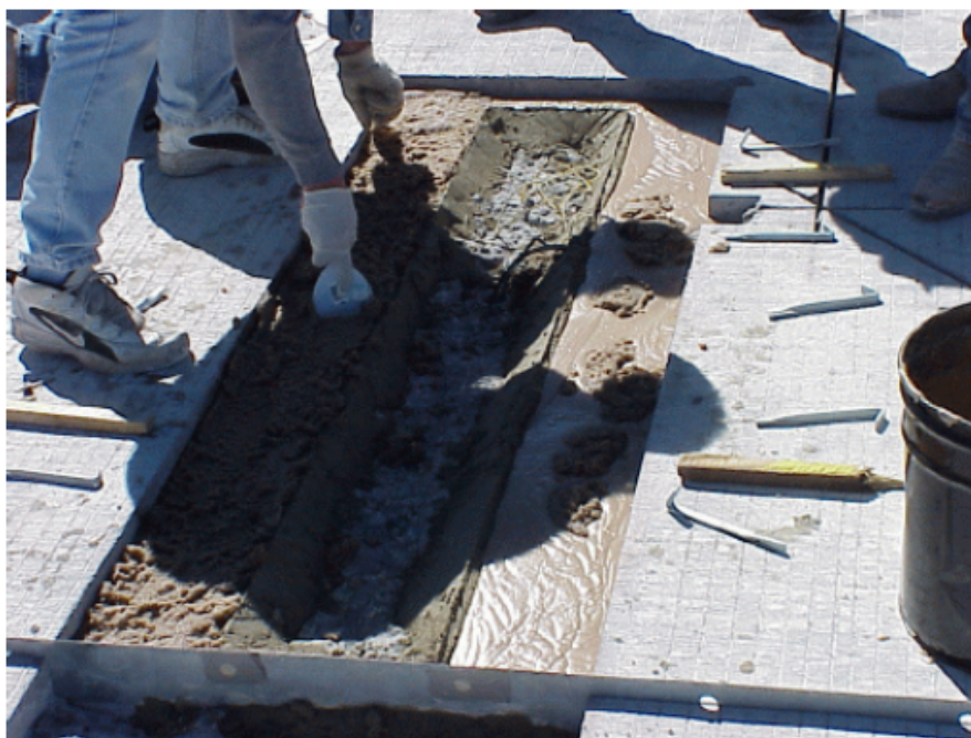
Figure 14 - Pouring Epoxy
