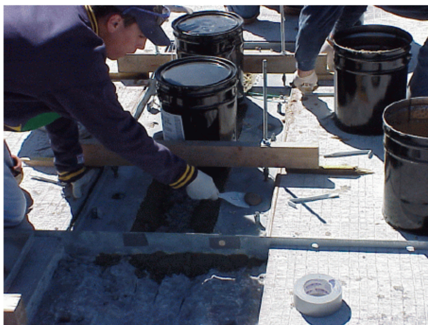
Figure 15 - Removing Excess Epoxy 123-429-901-000.jpg
