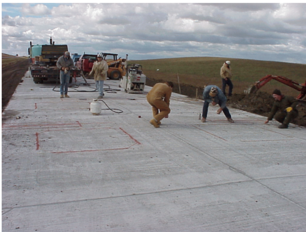
Figure 4 - Laying out Site
