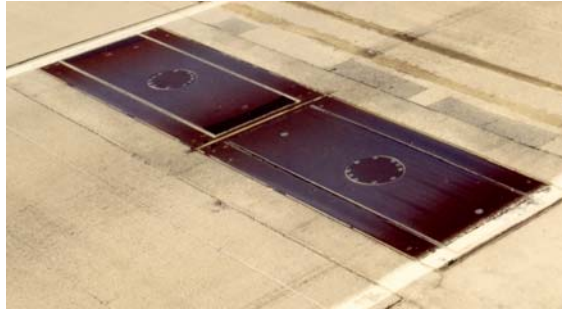
Figure 24 – Single Load Cell scales
