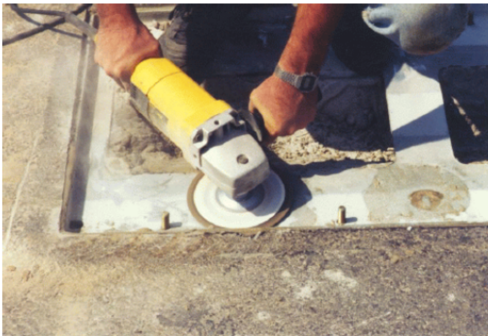
Figure 17 - Grinding Frame Clean
