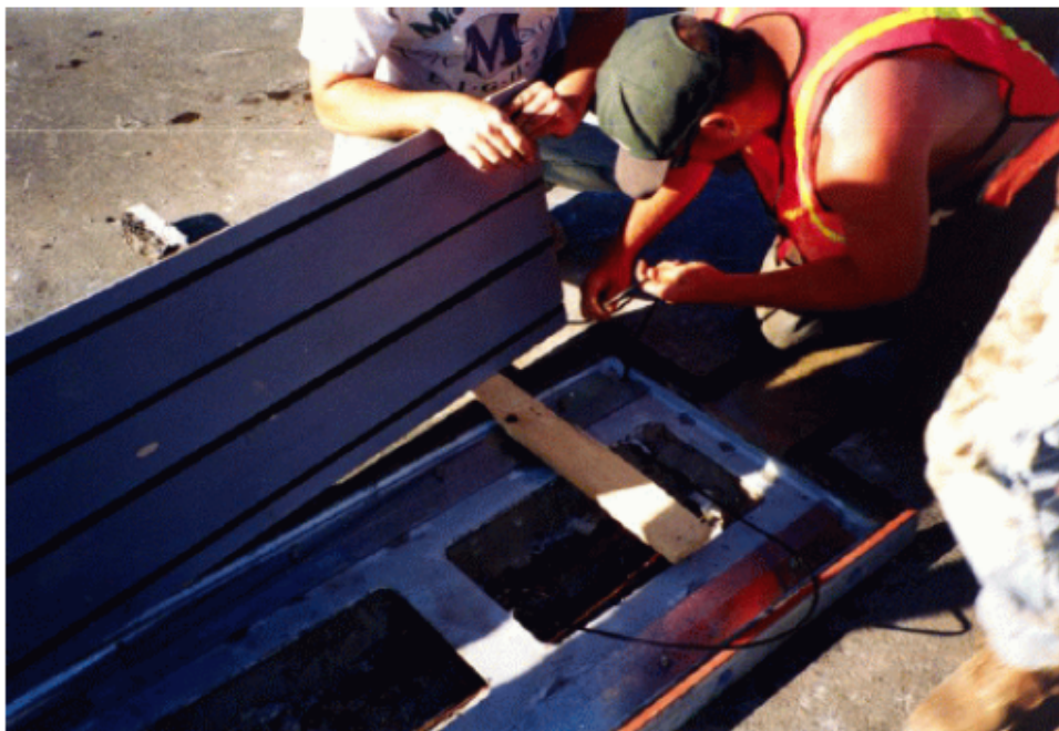
Figure 20 - Installing Weighpad
