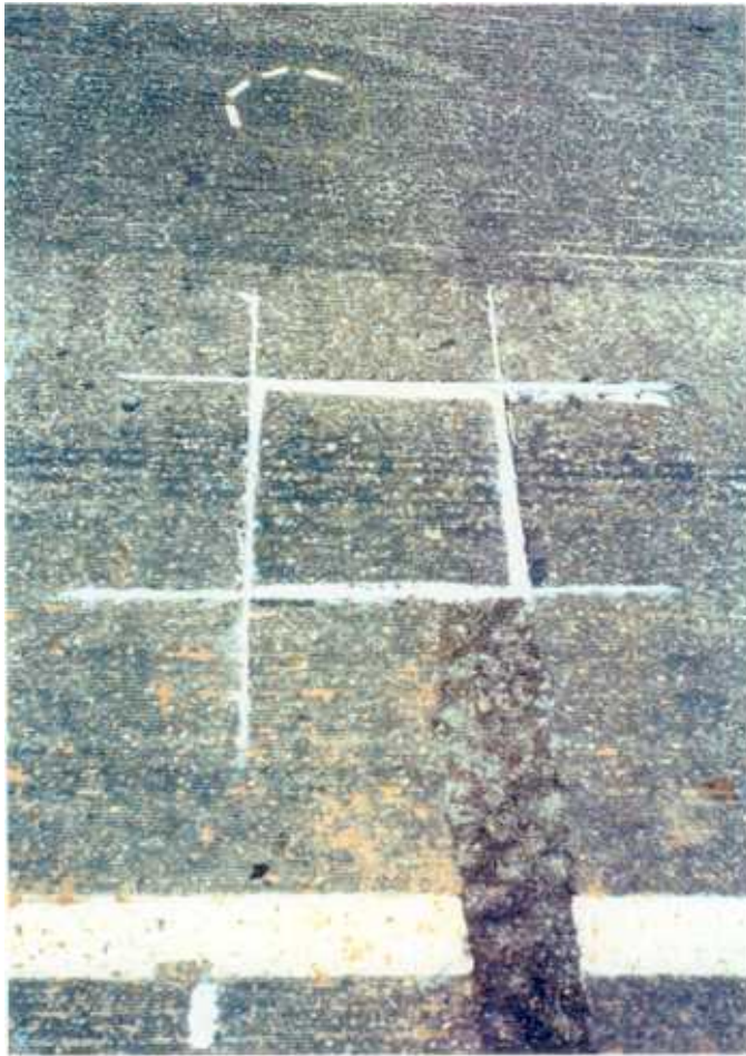
Photo E-7. Patched Instrumentation Area
