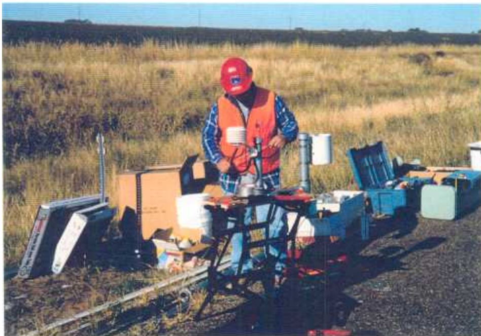
Photo E-6. Preparing Weather Station for Installation
