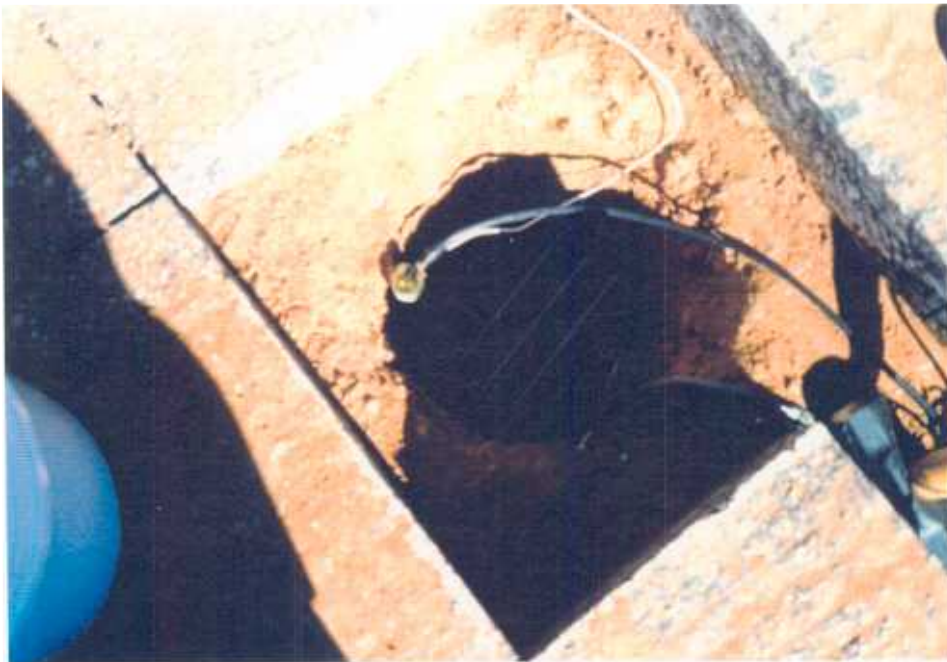
Photo E-4. Placement of Instrumentation Probes
