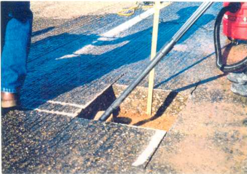
Photo E-3. Preparing for Instrumentation Installation
