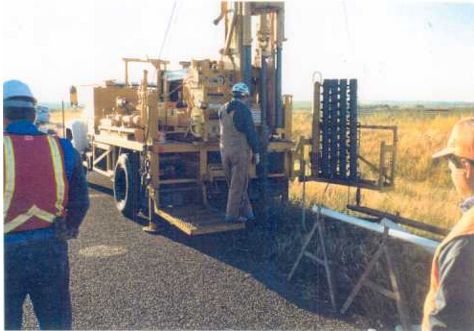
Photo E-5. Setting Monitoring Well
