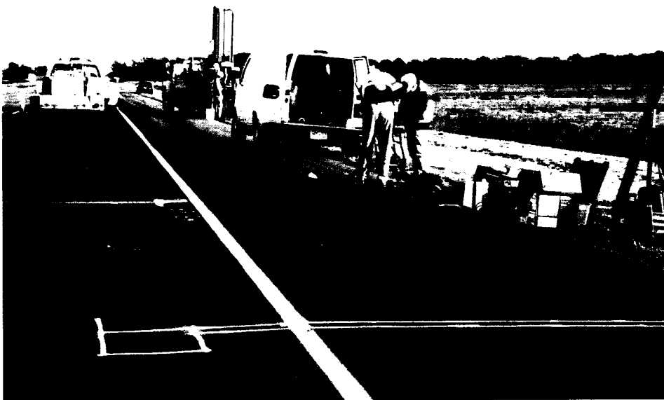
Photo E2 - Preparing Site for Installation
