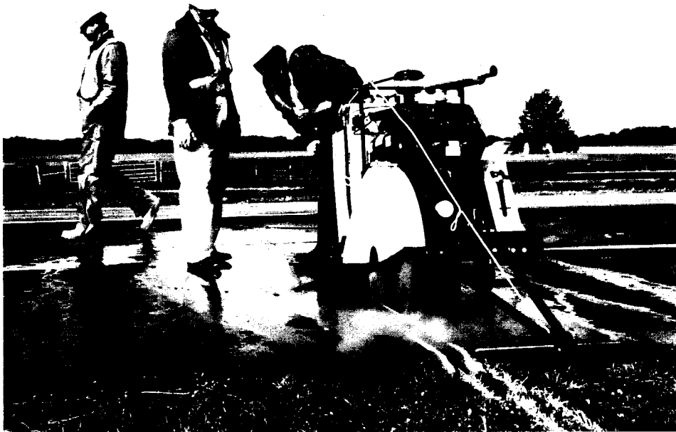
Photo E3 - Sawing Instrumentation Hole and Trench
