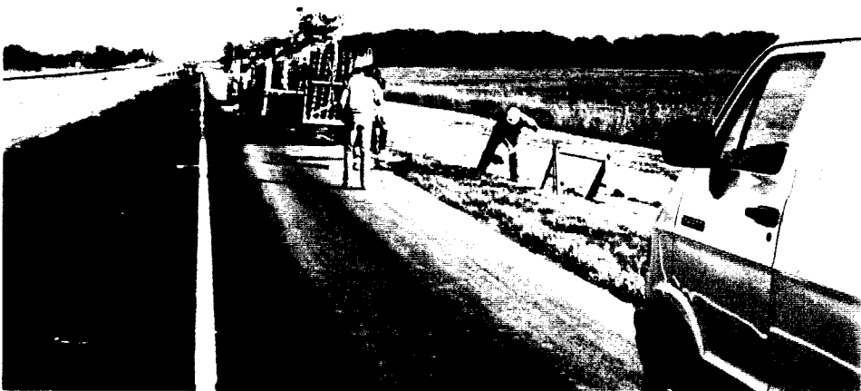
Photo E4 - Completion of Observation Well
