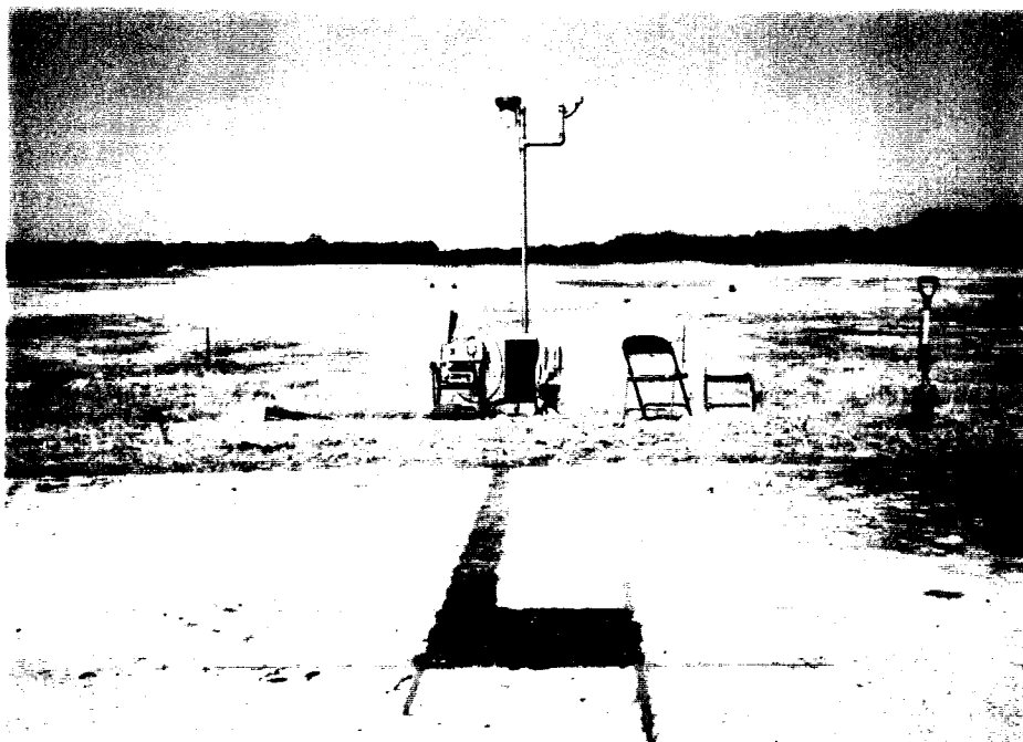
Photo E-4. Patched Instrumentation Area
