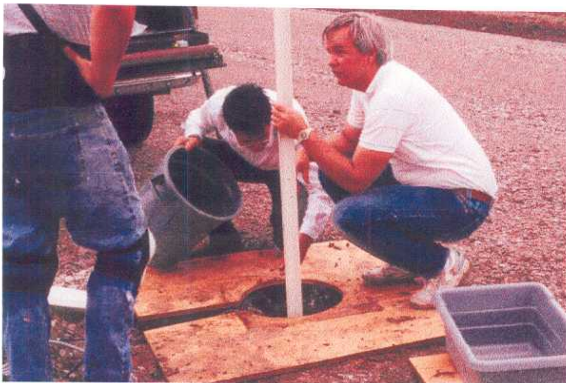
Photo 2 Compaction of backfill soil at Instrumentation Hole
