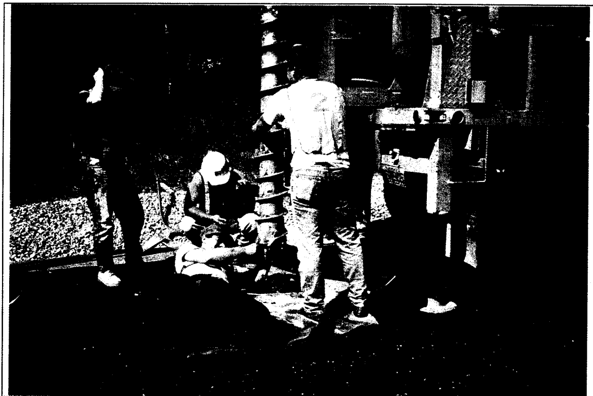
Figure E-1. Auguring the Instrument Hole, Section 370212, PATB in place, October 17, 1993
