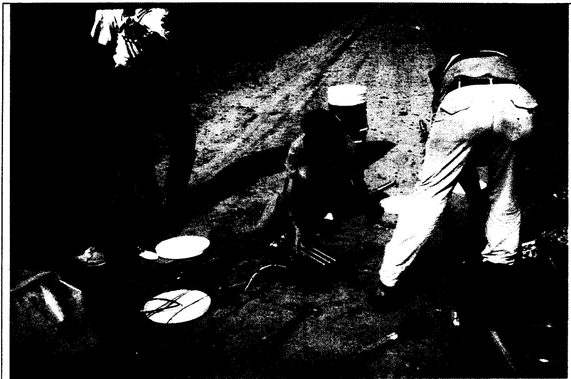
Figure E-4. Preparing top TDR for placement in DGAB layer (Section 370201), Oct. 17, 1993
