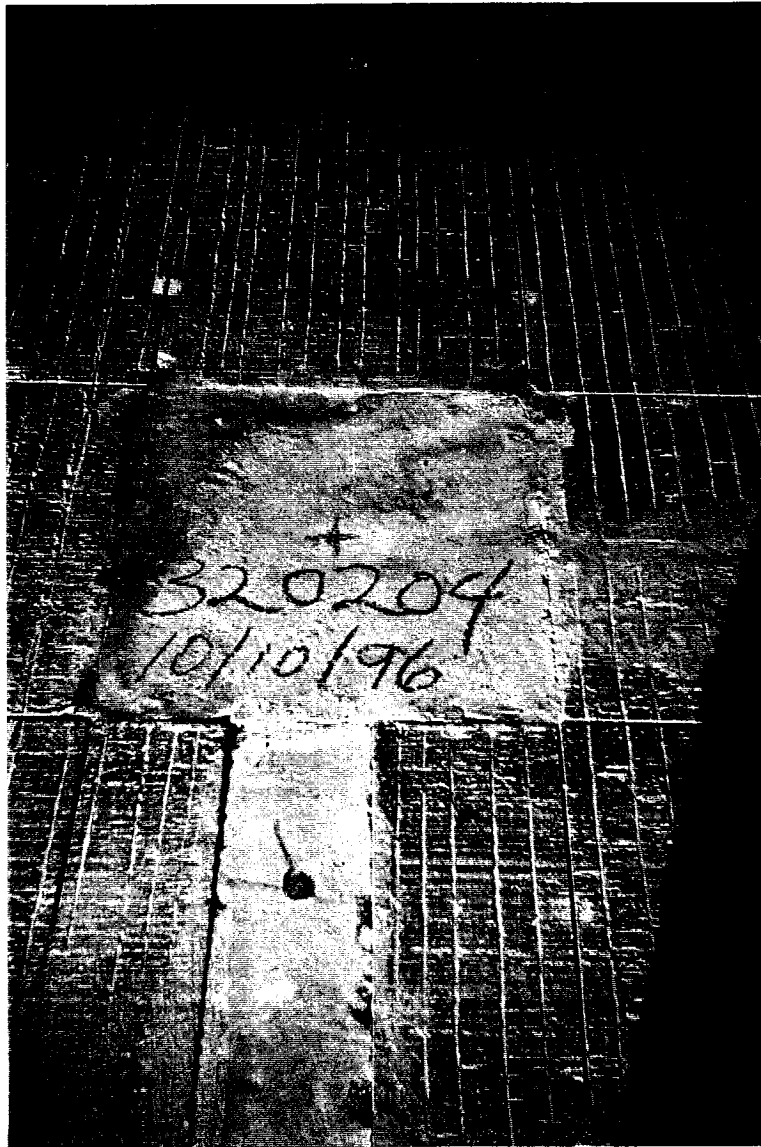
Figure C5. Instrumentation hole after repair.
