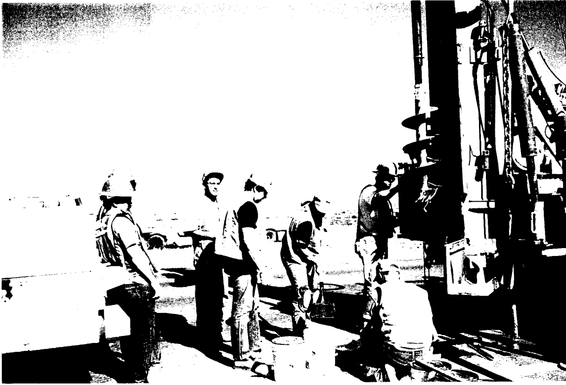
Figure C5. Instrumentation hole drilling in progress.
