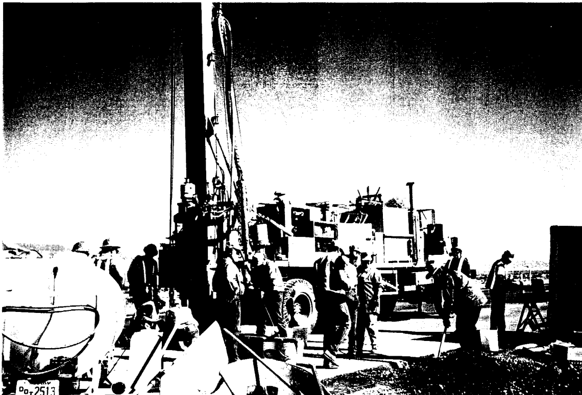
Figure C3. General activities during installation at the site.
