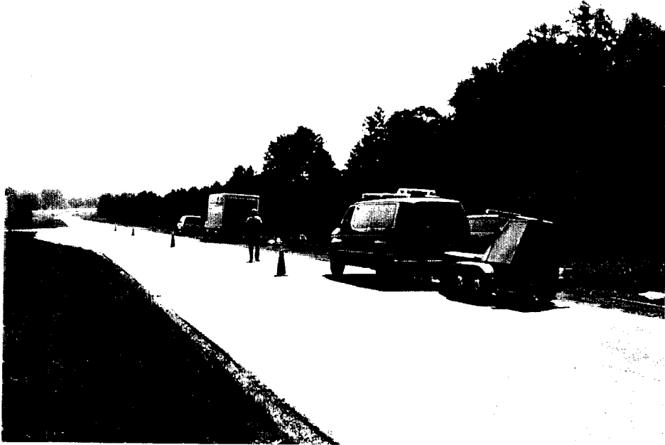
Photo E-1. FWD Testing Prior to Installation
