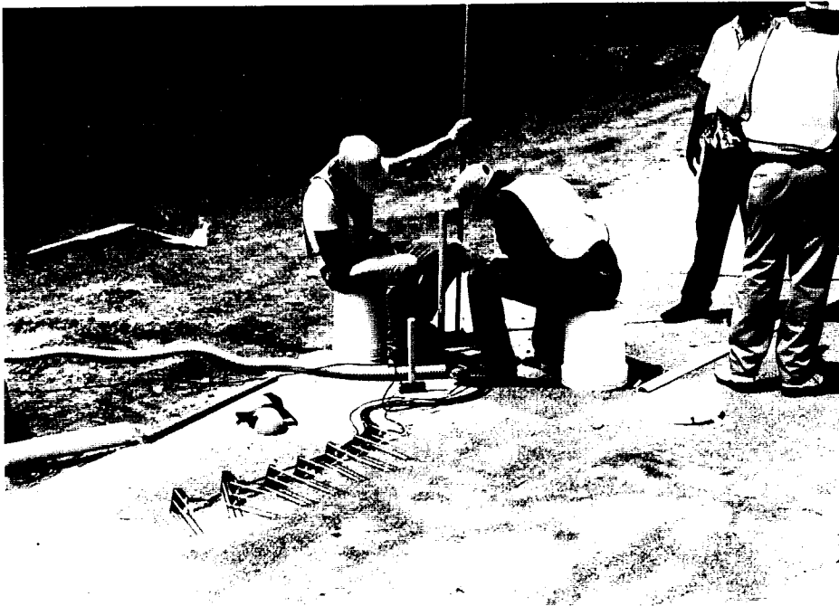
Photo E-4. Placement of TDRs During Backfilling of Soil
