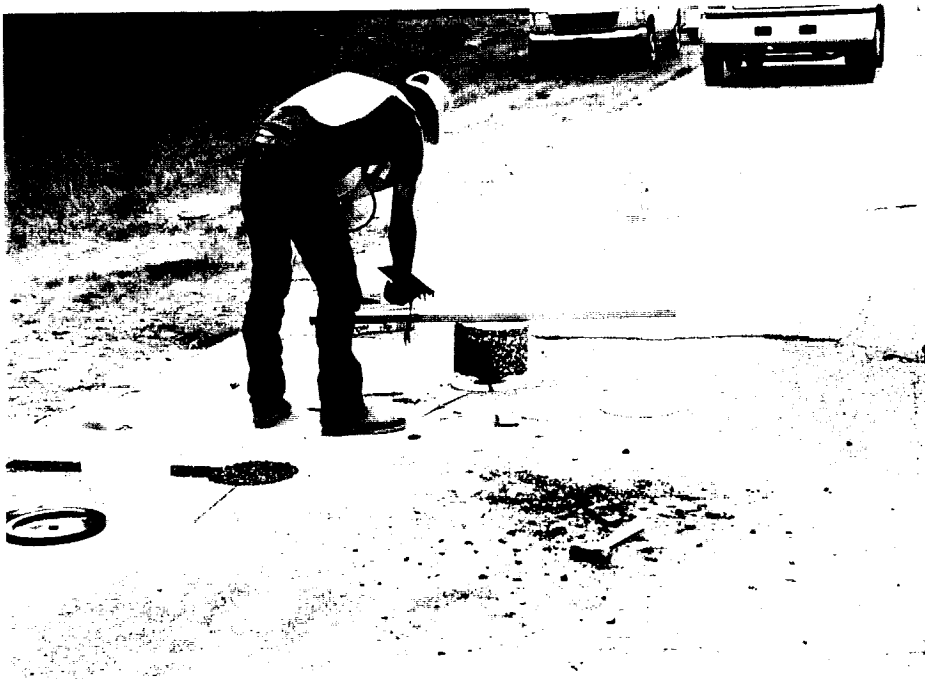
Photo E-5. Preparation of Core Prior to Replacement
