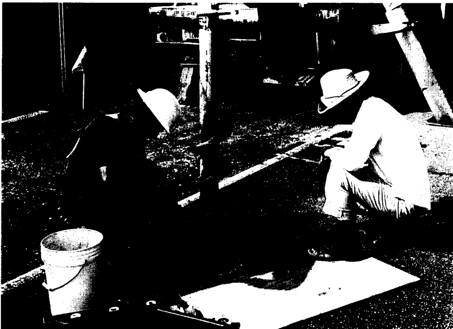
Photo E-2. Augering of Instrumentation Hole
