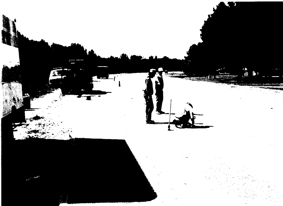
Photo E-1. Setting PK Nails to Mark Test Section
