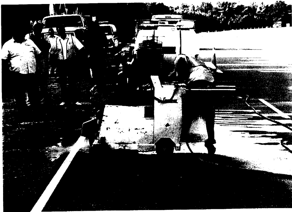
Photo E-3. Cutting of Trench with Pavement Saw
