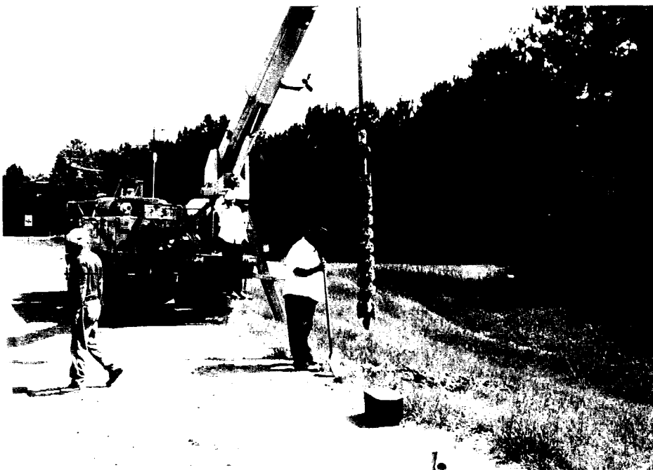
Photo E-2. Augering of Piezometer Observation Well
