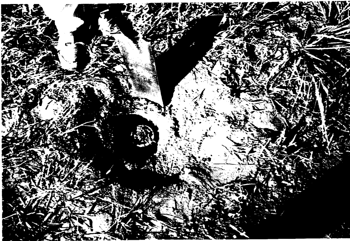
Photo E-3. Installation of Piezometer Observation Well
