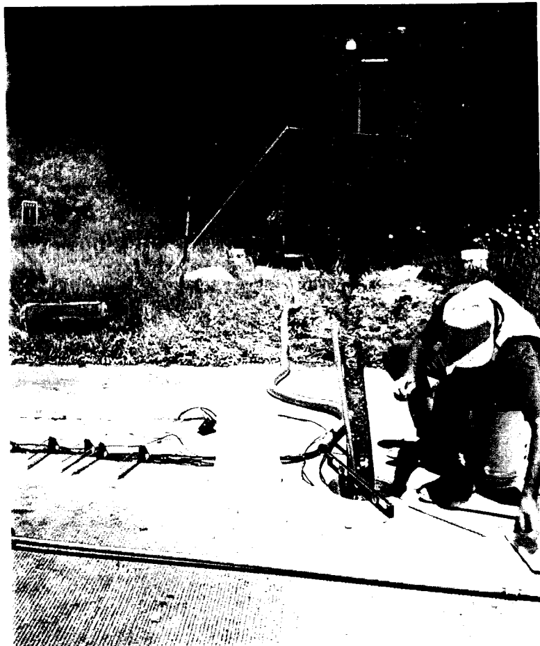
Photo E-4. Preparing for Instrumentation Installation
