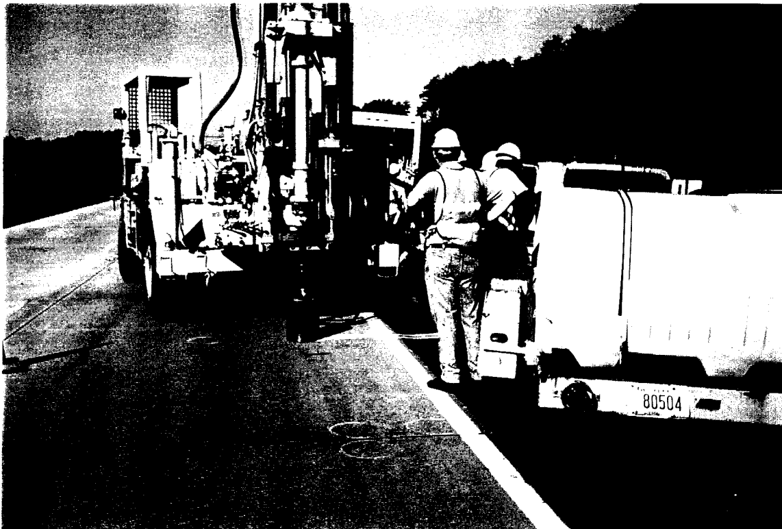
Photo E-2. Removal of Pavement Core
