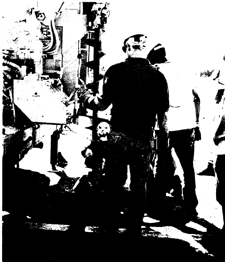
Photo E-1. Operation of Auger Rig
