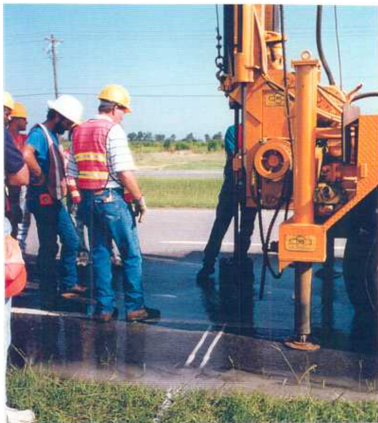
Photo E-2. Removal of Pavement Core
