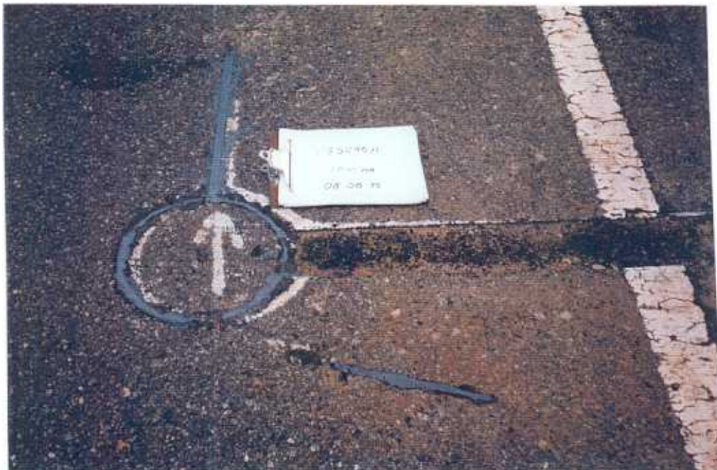
Photo E-4. Final Core Replacement and Sealant
