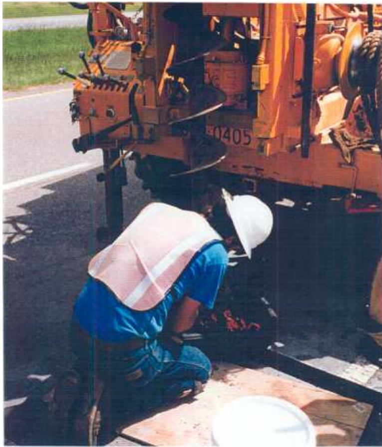
Photo E-3. Removal of Soil from Instrumentation Hole
