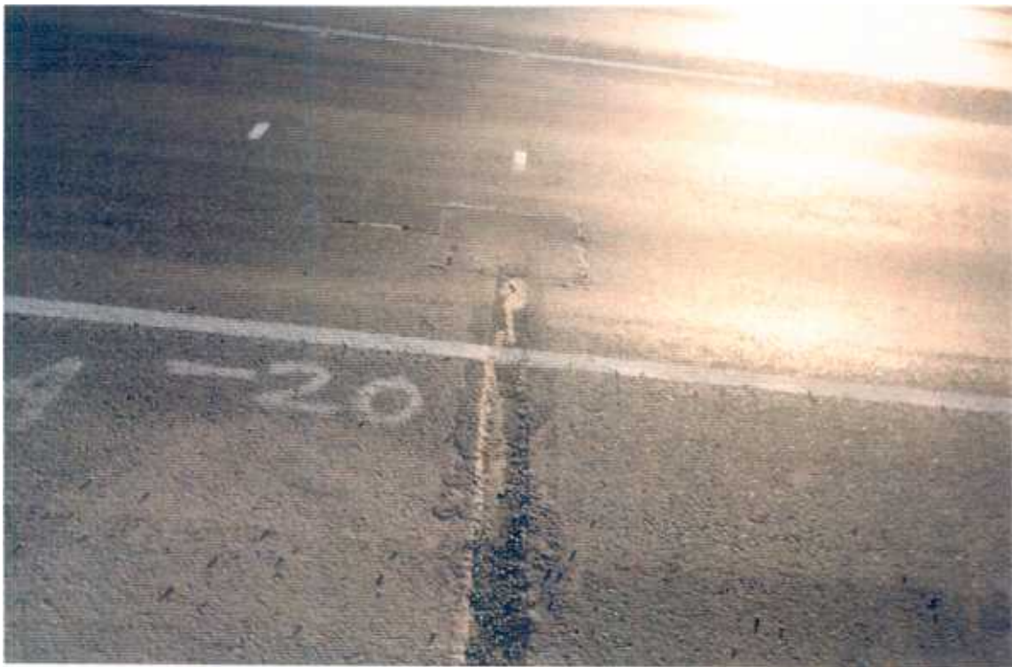
INSTRUMENTATION TRENCH FEBRUARY 1995
