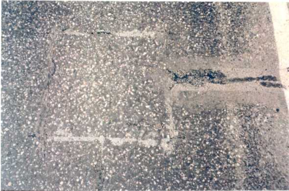
INSTRUMENTATION HOLE JANUARY 1995
