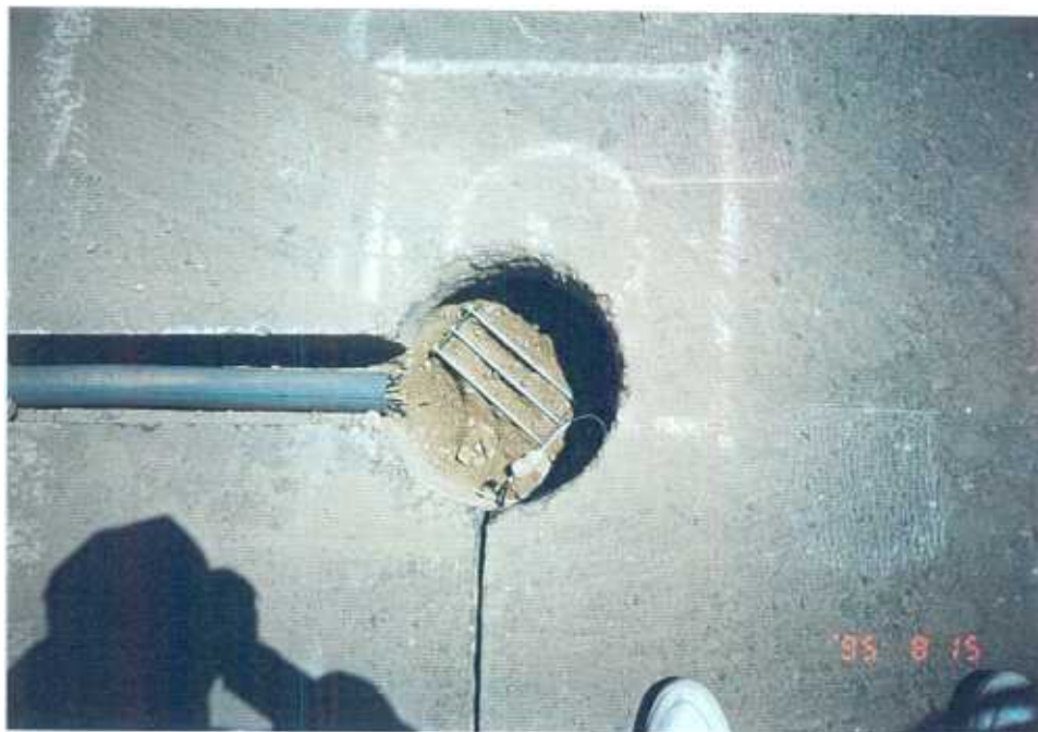
Figure C5. Instrument installation in progress.
