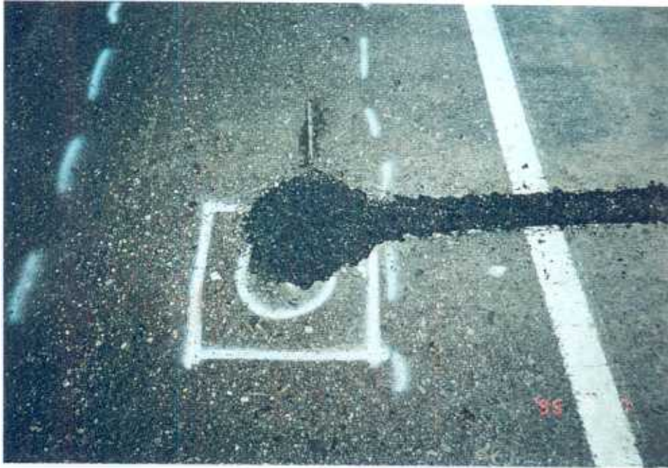
Figure C7. Instrumentation hole after repair.
