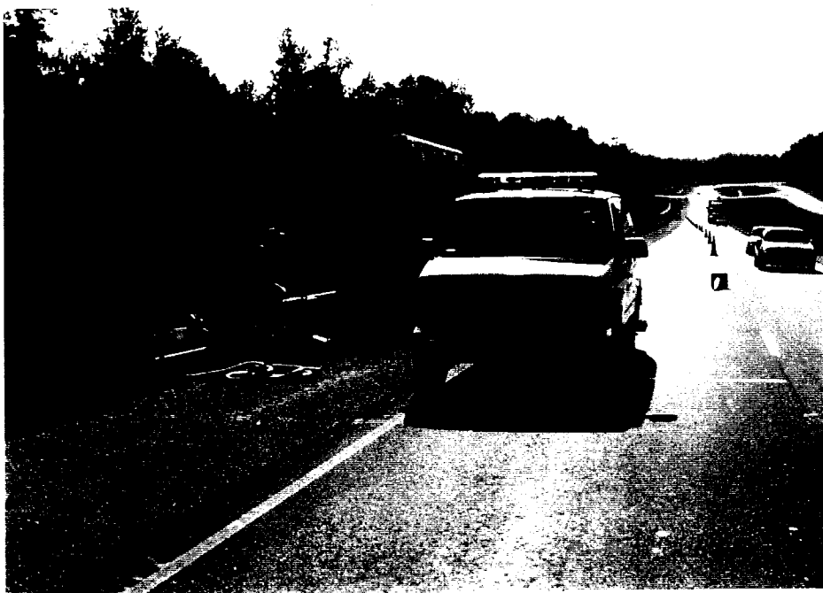
Photo E-1. Falling Weight Deflectometer (FWD) Testing Prior to Installation
