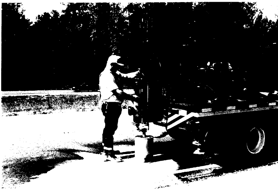
Photo E-2. Cutting of Pavement Core Over Instrumentation Site
