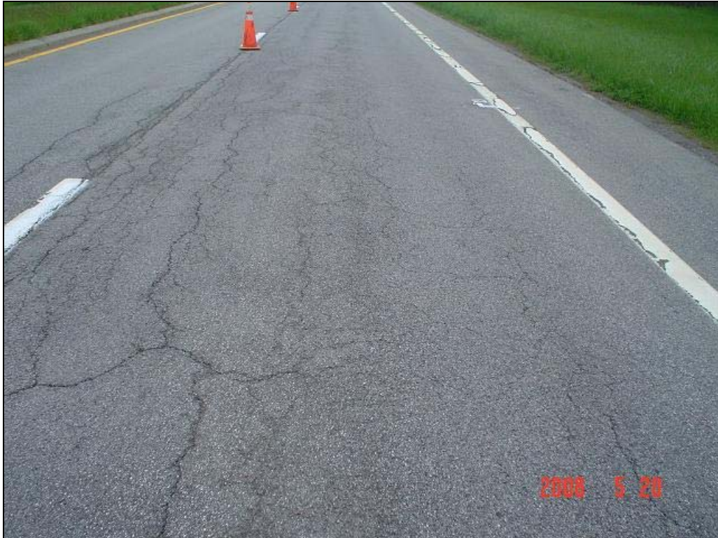
Figure E-3: Photo of Multiple Cracks in Vicinity of Station 1+00 (360801)
