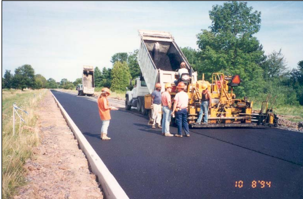
D-5: Placement of Asphalt Base Layer – Section 360801 Driving Lane (Blaw-Knox model CPF-200 AP87 Paver)
