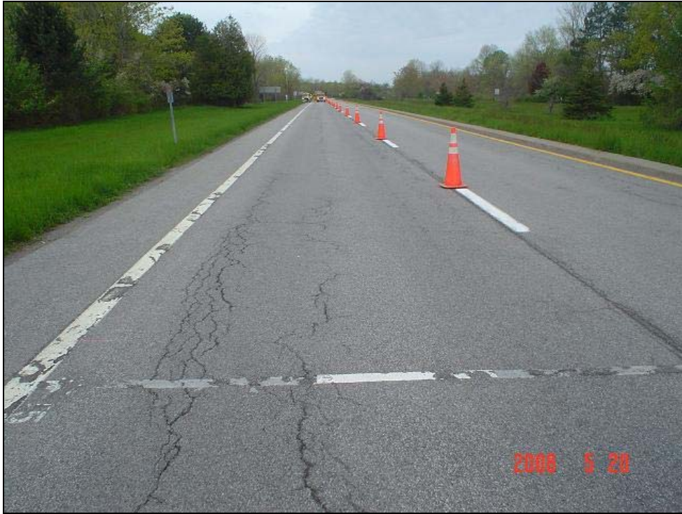
Figure E-5: Photo of Moderate Severity Alligator Crack in Outer Wheel Path (360801)
