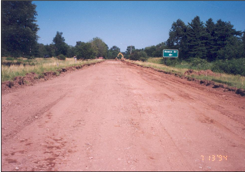
Figure D-1: Subgrade Preparation Looking East - Section 360801 to 360802
