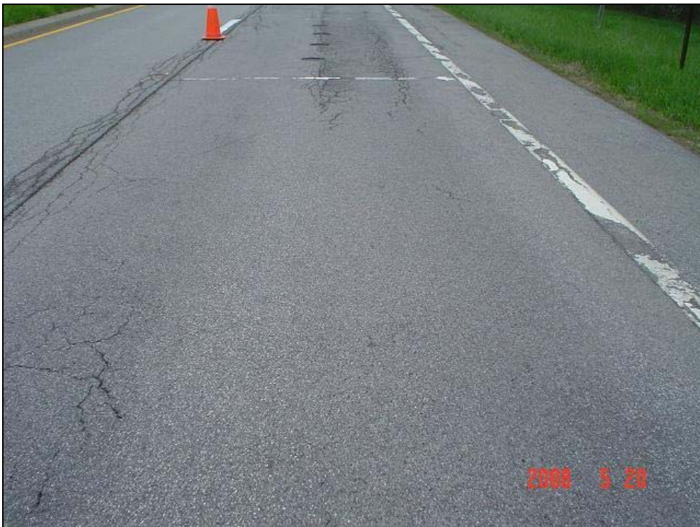
Figure E-10: Photo of High Severity Cracking/Ravelling from End of Section towards Core Sample Locations Station 5+00 (360802)
