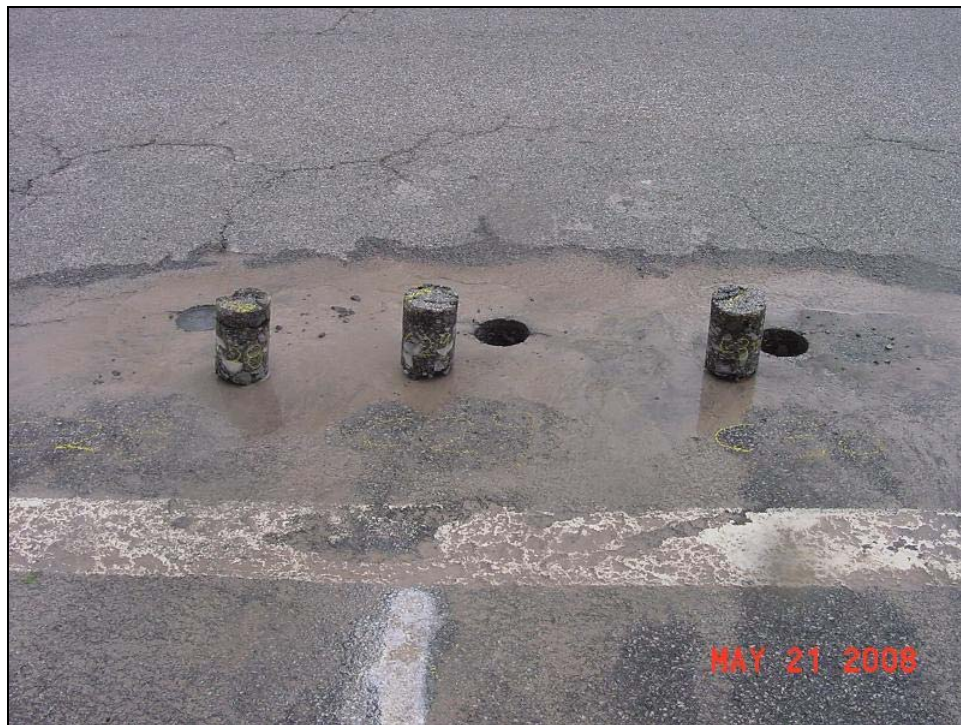
Figure F-8: 100mm Cores at Alligator Cracks in Outer Wheel Path (360801)
