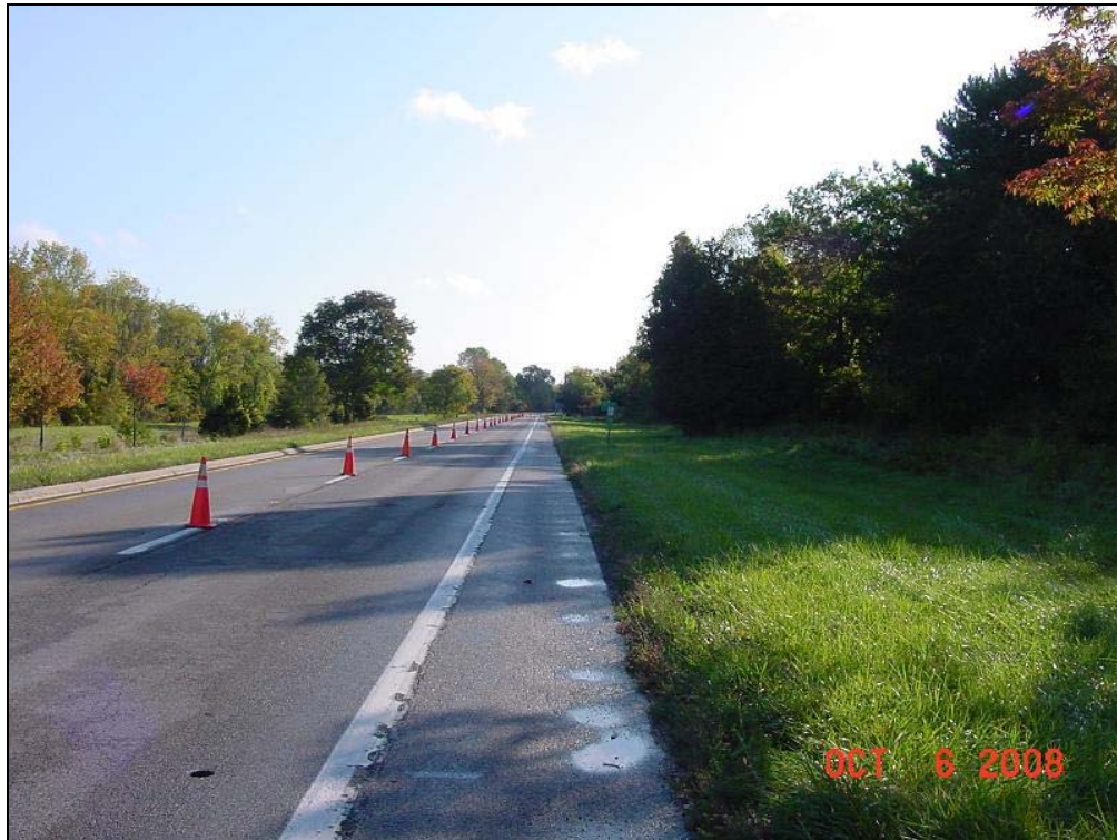
Figure E-12: Photo of Shoulder with Turf Grade Higher Than AC (360801)
