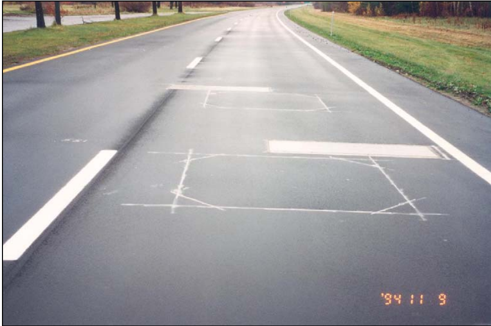
Figure E-1: Weigh-in-Motion (WIM) Installed at SPS-8 Project
