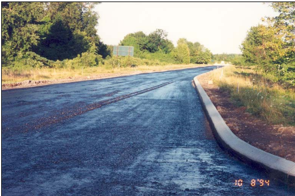
Figure D-4: Tack Coat Applied to Finished Aggregate Base Looking West – Section 360802 to 360801
