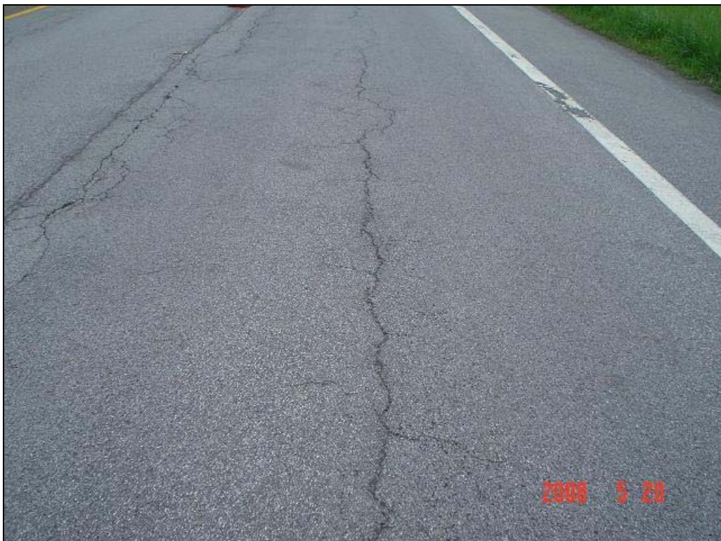
Figure E-4: Photo of Mid-Lane Longitudinal with Associated Cracking (360801)
