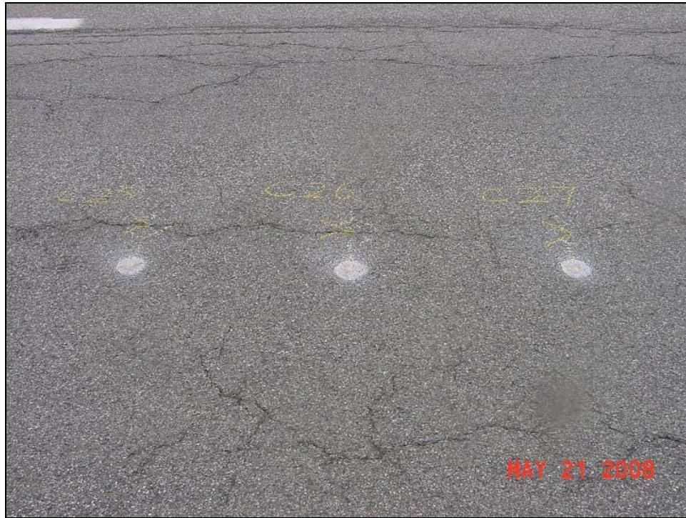
Figure F-1: Core Location Marking at a Midlane Longitudinal Crack (360801)
