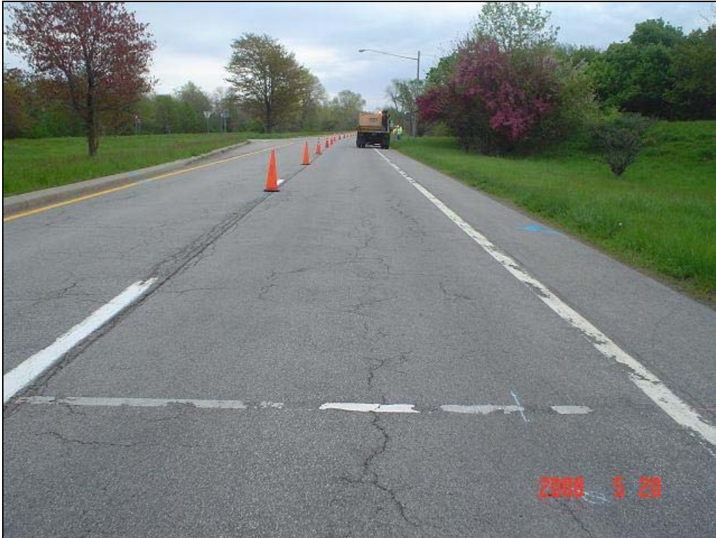
Figure E-7: Photo of Multiple Random Cracking at Station 0+00 (360802)
