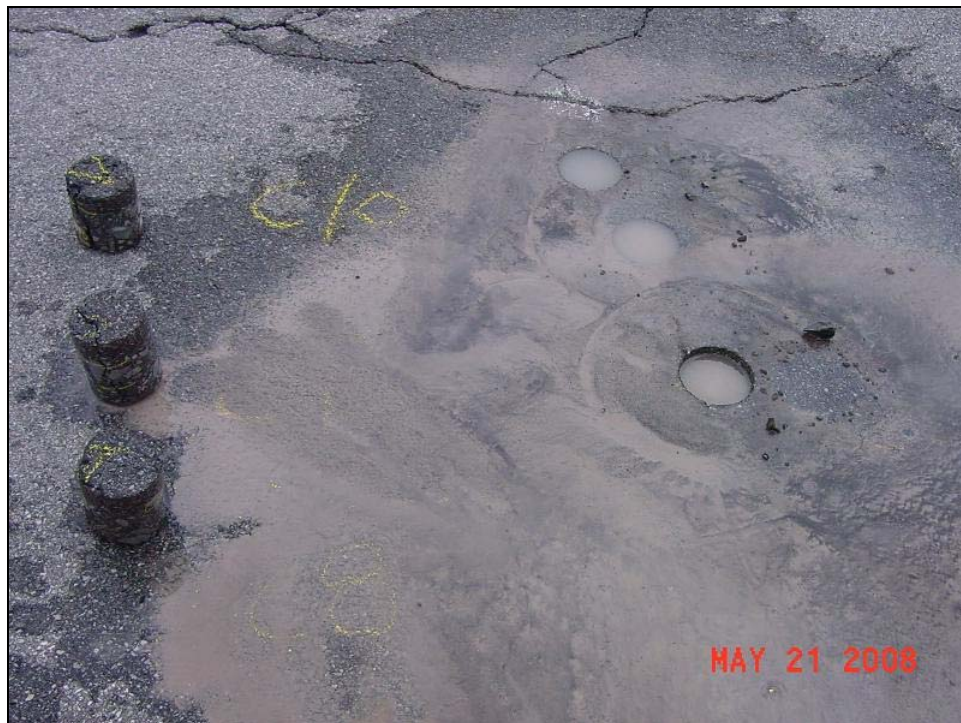
Figure F-4: 100mm Cores at Partial Transverse Crack (360801)
