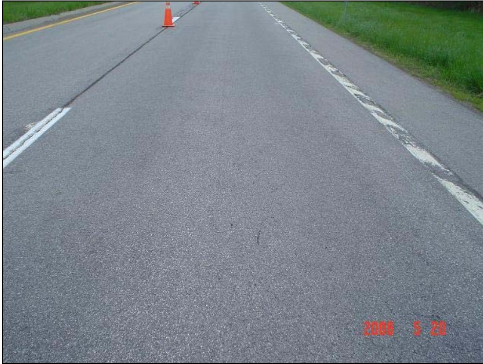
Figure E-9: Photo of Low Severity Alligator Cracks in Wheel Paths (360802)
