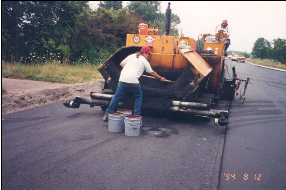
Figure D-7: Obtaining Asphalt Samples for Laboratory Analysis and Shipment to the FHWA-LTPP Materials Research Library (MRL)
