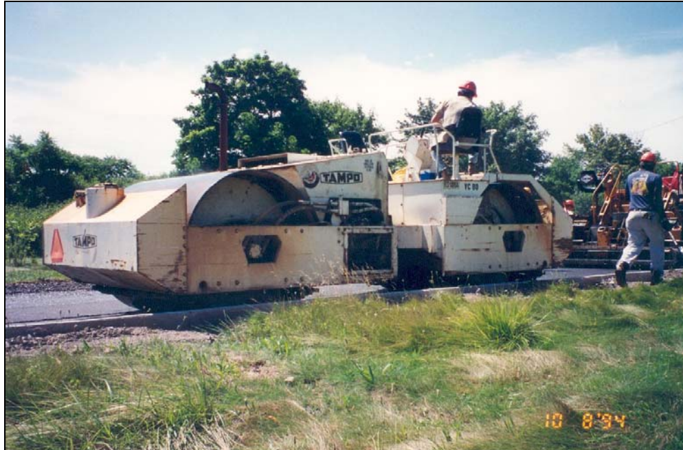
D-6: Compaction of Asphalt Base Layer (Tampon RS-188A Model VC80 Double-Drum Vibratory Roller)
