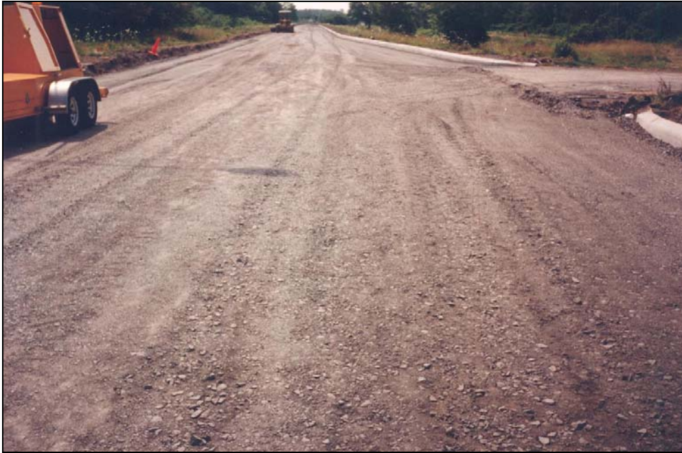
Figure D-3: FWD Testing and Fine Grading of Aggregate Base Looking West - Section 360802 to 360801
