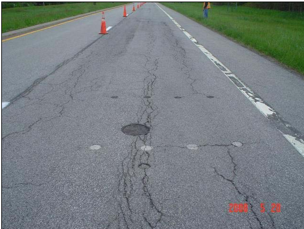
Figure E-6: Photo of High Severity Distress between Section 360801 and 360802
