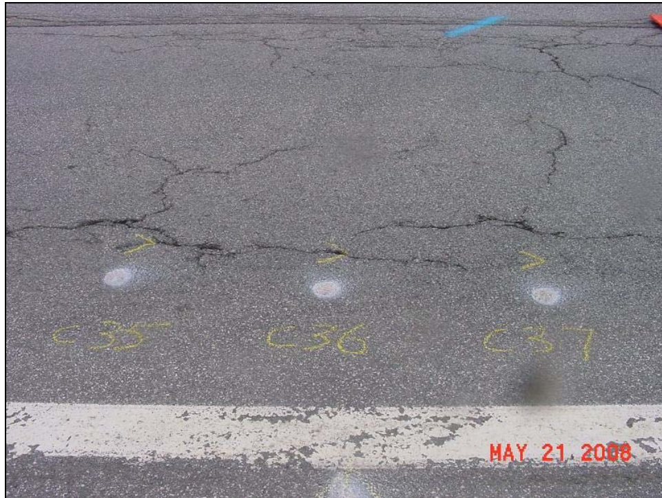
Figure F-9: Marks Identifying Location for Cores in Outer Wheel Path (360802)
