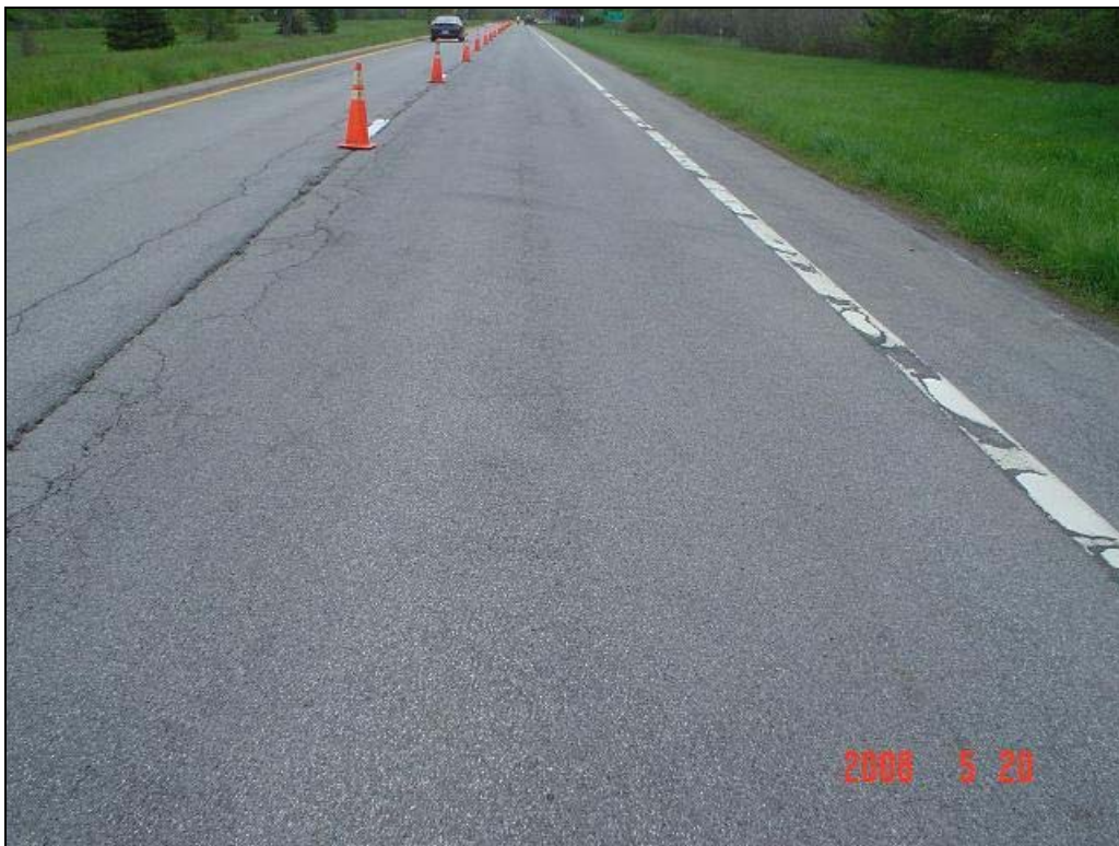
Figure E-2: Photo of High Severity Centerline Longitudinal Crack with Associated Cracking (360801)
