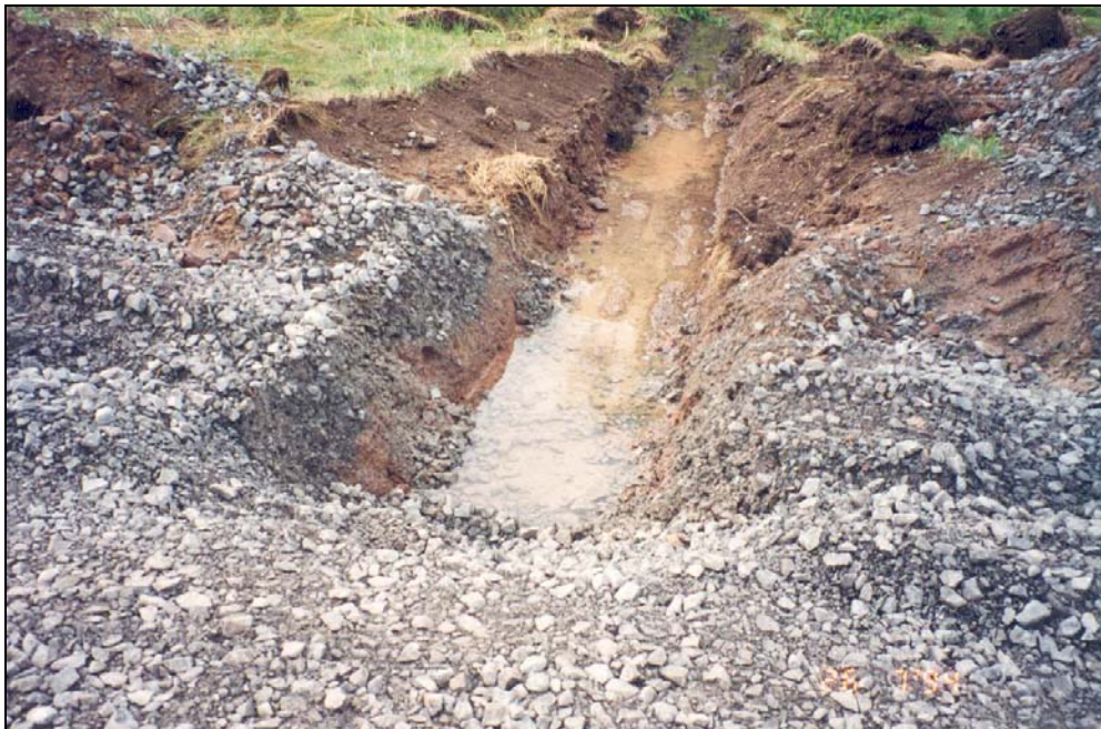
Figure D-2: Trenching to Remove Moisture from Base/Subgrade Material during Construction of Section 360801
