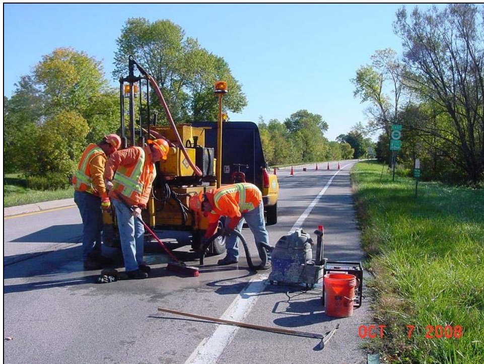
Figure F-2: NYSDOT coring - 100mm and 150mm Cores
