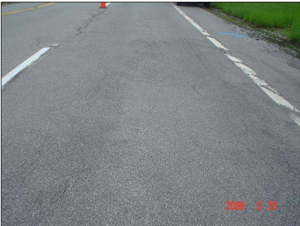
Figure E- 8: Photo at Location of Water Utility – Signs of Leakage (360802)
