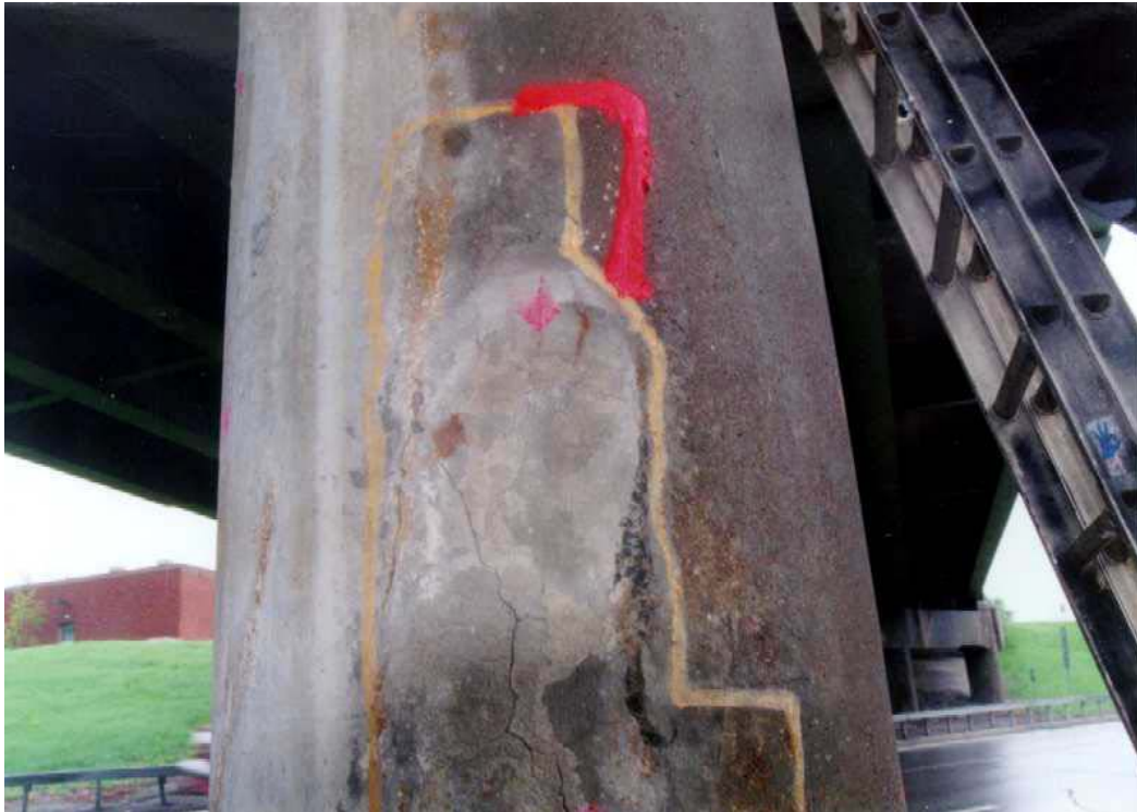
Figure 42. Photo. First view of a completely delaminated patch (marked in yellow) on a column of the Campus Loop Bridge in Albany, NY.
