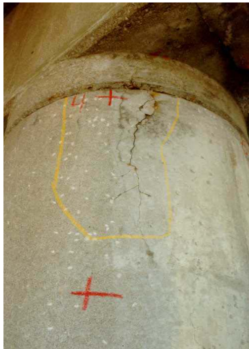
Figure 40. Photo. Cracks and rust staining in a nonpatched area of a column of the Campus Loop Bridge in Albany, NY, during the second visit in 1996.
