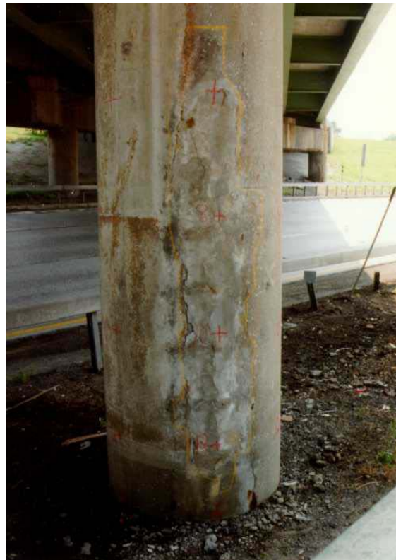
Figure 38. Photo. First view of cracks and rust staining in patched and nonpatched areas of the columns of the Campus Loop Bridge in Albany, NY, during the second visit in 1996.
