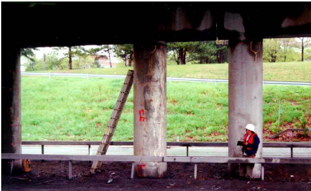
Figure 41. Photo. Water flowing down the pier caps and columns through leaking joints.
