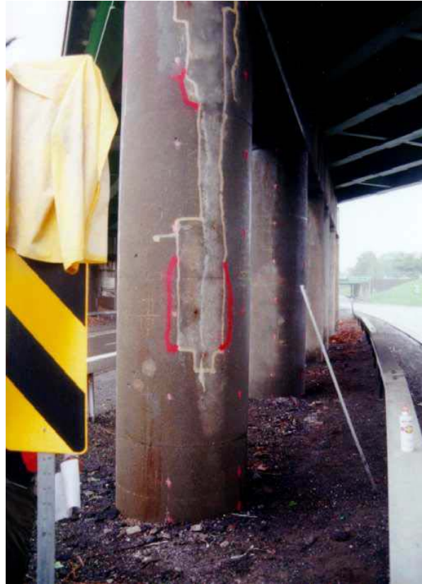
Figure 43. Photo. Second view of a completely delaminated patch (marked in yellow) on a column of the Campus Loop Bridge in Albany, NY.
