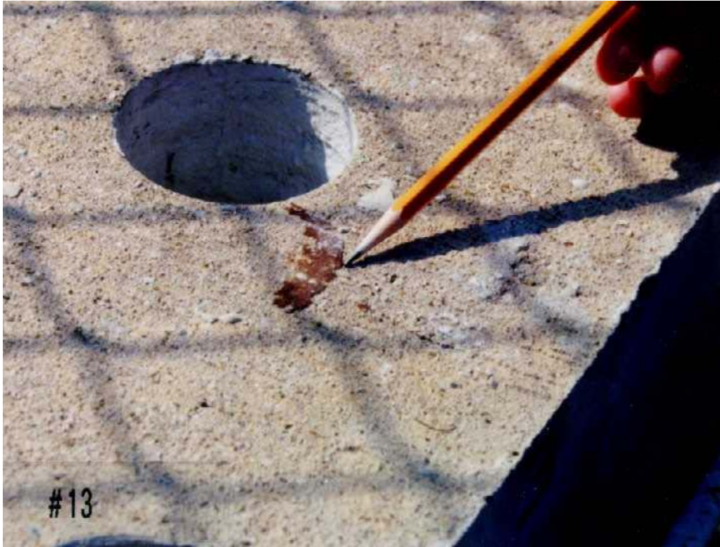
Figure 14. Photo. Rust staining on the top surface of slabs 3 and 4.
