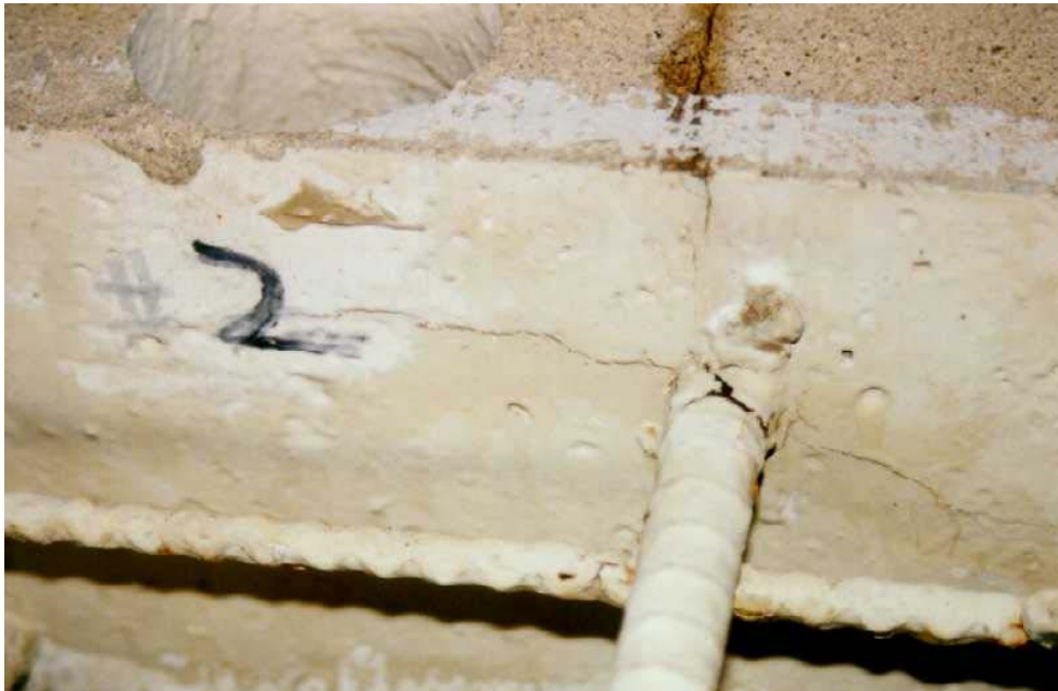
Figure 5. Photo. Termination of the top crack and other cracks on the front side of slab 2 in August 1994.
