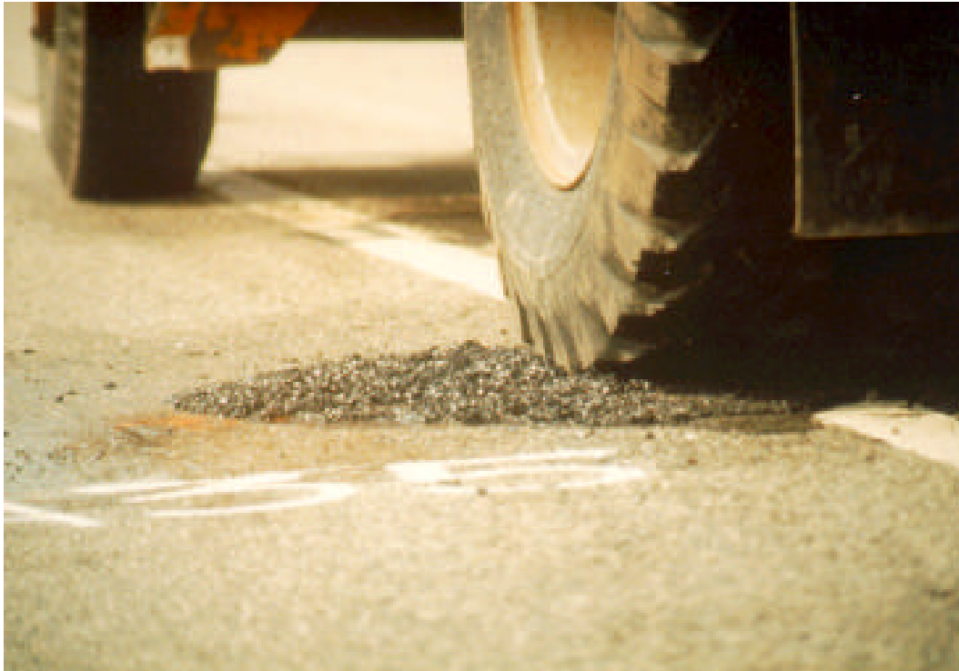
Figure 2. Throw-and-roll procedure—compaction of patch.
