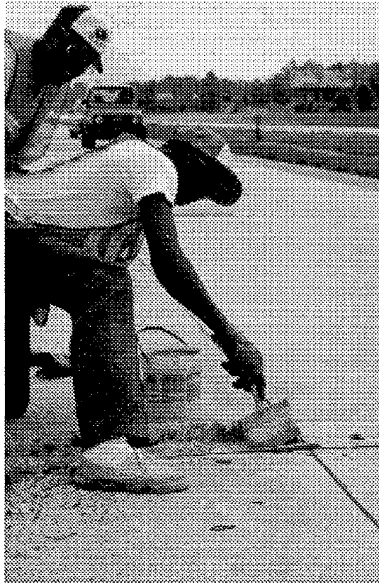
Figure 12. Application of epoxy bonding agent.
