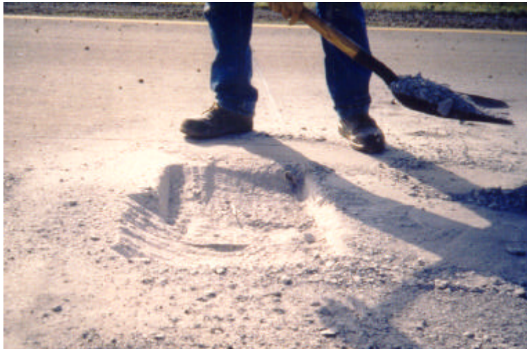
Figure 7b. Milled patch with rounded edges.
