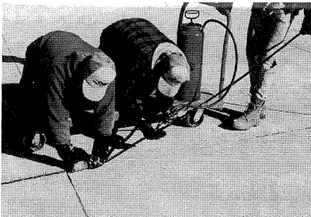
Figure 21. Manual installation of neoprene compression seal at Tremonton, Utah test site.
