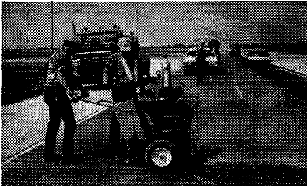
Figure 17. Random crack saw with 200-mm diamond blade.
