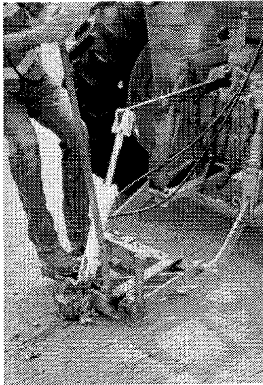
Figure 10. Joint plowing operation.
