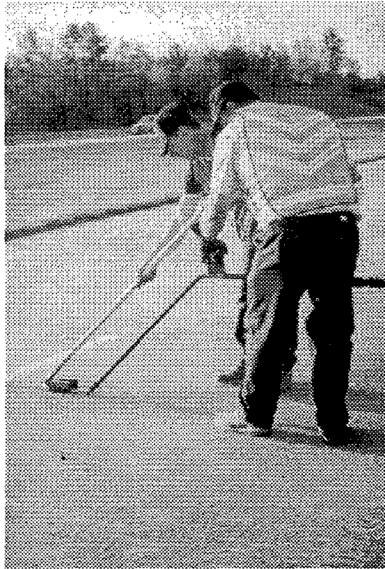
Figure 18. Overbanded sealant installation.
