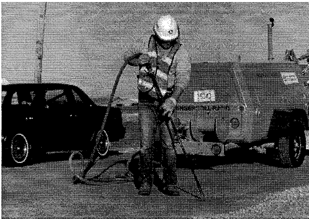
Figure 14. Airblasting operation.
