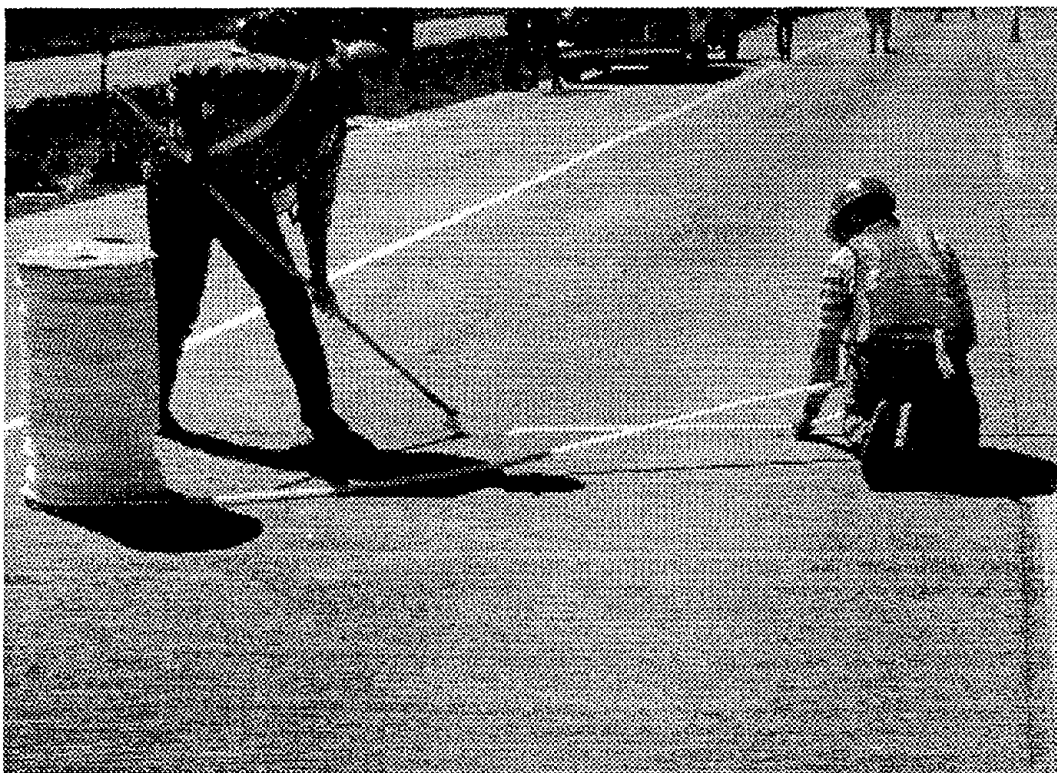
Figure 15. Backer rod installation.
