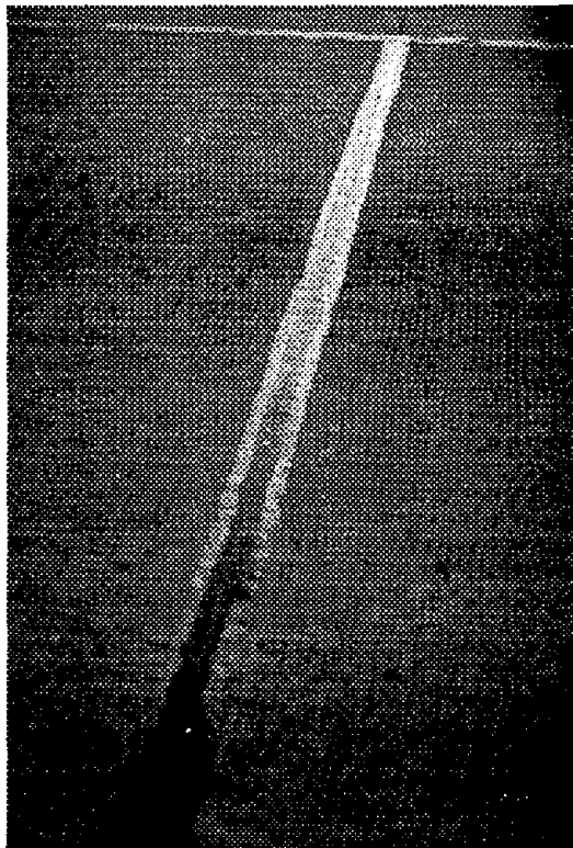
Figure 18. Overbanded sealant installation.
