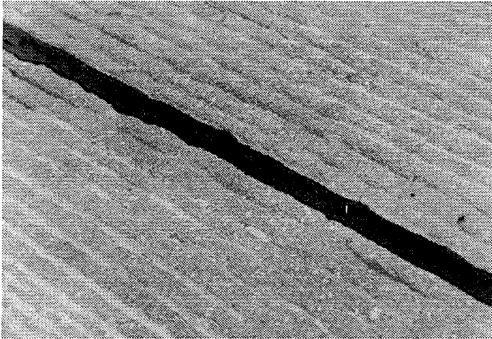
Figure 17. Installed flush-filled sealant.
