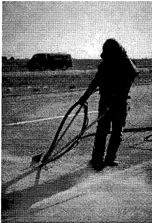
Figure 13. Sandblasting operation.
