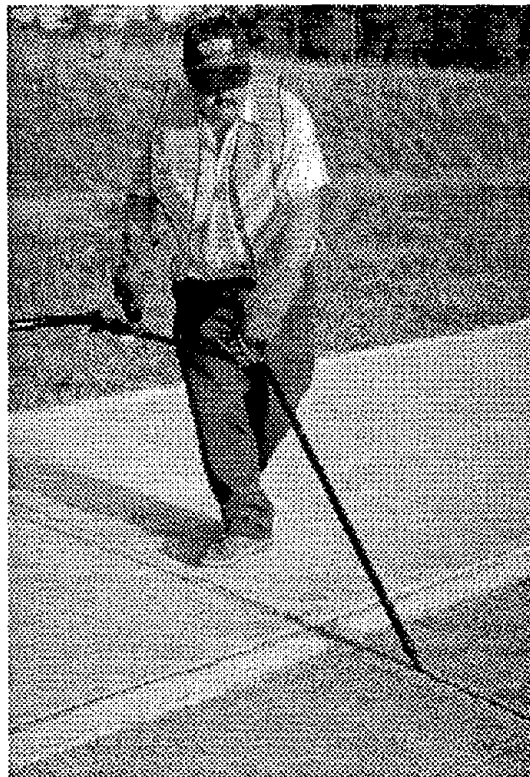
Figure 16. Recessed sealant installation.
