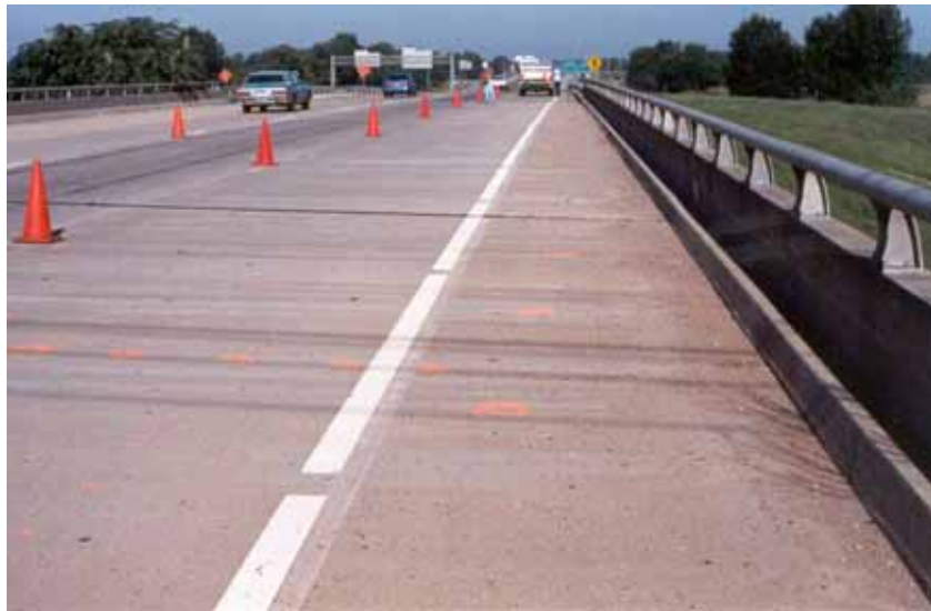
Figure 17. Photograph of I-265 northbound lanes with latex-modified overlay.
