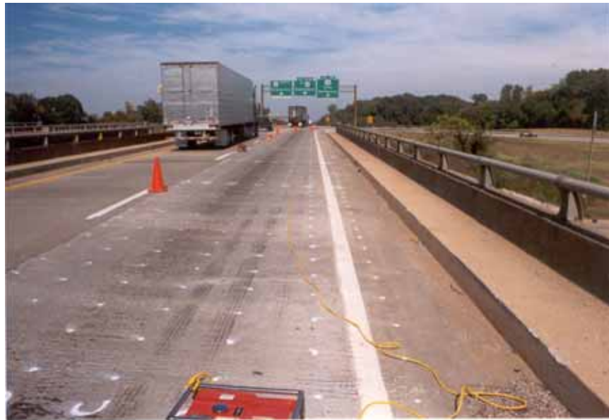
Figure 23. Photograph of northbound test section of U.S. 41 (latex-modified concrete overlay).
