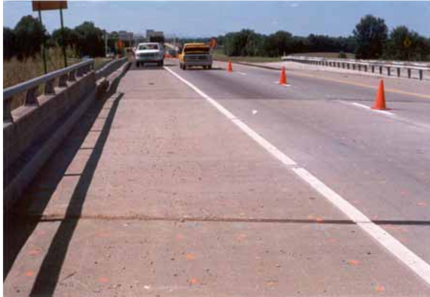
Figure 18. Photograph showing I-265 southbound lanes with silica fume concrete overlay.
