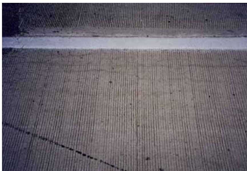
(i) Control section 5 (C5)
