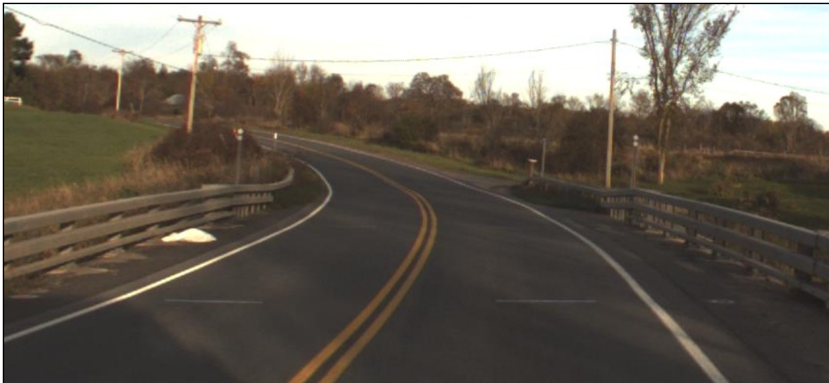
Figure 19. Photo. A GRS-IBS bridge in St. Lawrence County, NY (eastbound direction).
