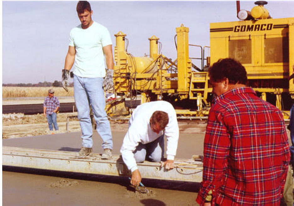
Figure 12.14 Pulling Protective Boxes
