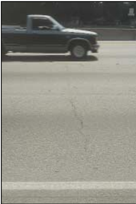
FIGURE 19 Distress Type ACP 6—Low Severity Transverse Cracking
