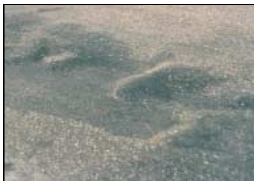
FIGURE 35 Distress Type ACP 10—Shoving in Pavement Surface
