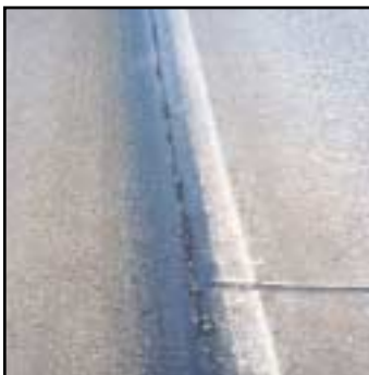
FIGURE 82 Distress Type JCP 14—Poorly Sealed Lane-to-Shoulder Separation
