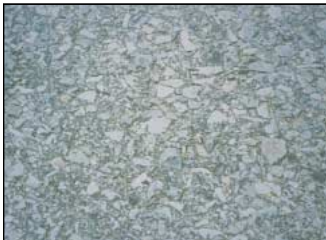
FIGURE 39 Distress Type ACP 12—Polished Aggregate
