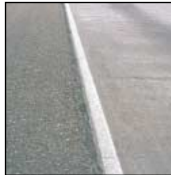
FIGURE 83 Distress Type JCP 14—Well-Sealed Lane-to-Shoulder Separation
