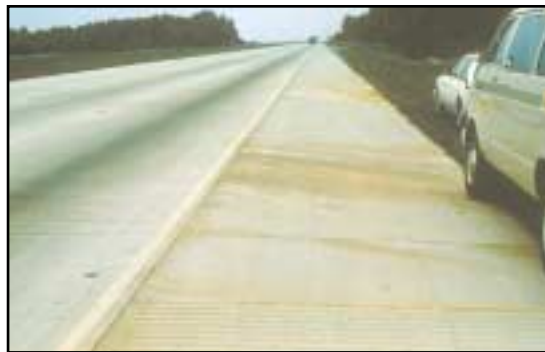
FIGURE 131 Distress Type CRCP 14—Water Bleeding and Pumping
