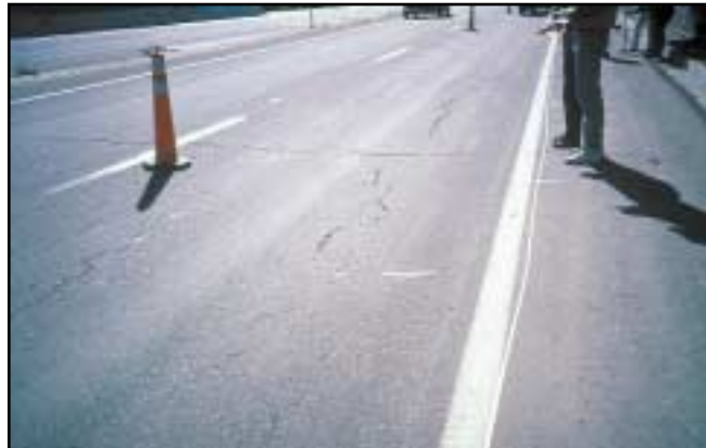
FIGURE 5 Distress Type ACP 1—Low Severity Fatigue Cracking
