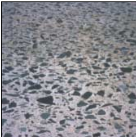
FIGURE 72 Distress Type JCP 9—Polished Aggregate
