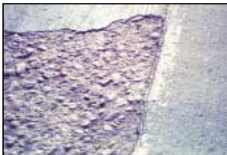
FIGURE 70 Distress Type JCP 8b—Scaling
