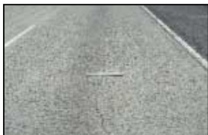
Figure 94 Distress Type CRCP 2—Low Severity Longitudinal Cracking
