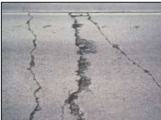
FIGURE 100 Distress Type CRCP 3—High Severity Transverse Cracking
