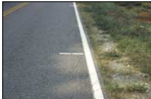
FIGURE 12 Distress Type ACP 3—Low Severity Edge Cracking
