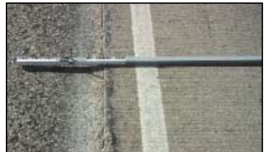
FIGURE 80 Distress Type JCP 13— Lane-to-Shoulder Dropoff
