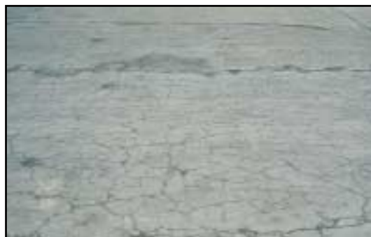
FIGURE 69 Distress Type JCP 8a—Map Cracking
