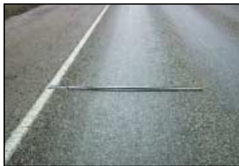
FIGURE 32 Distress Type ACP 9—Rutting
