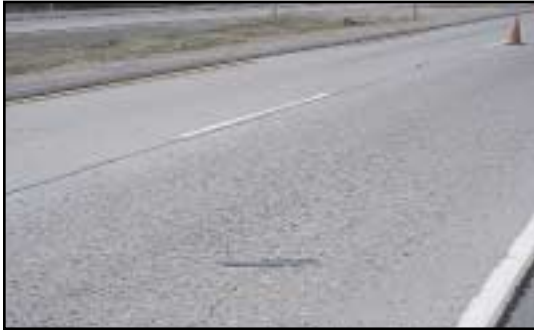
FIGURE 55 Distress Type JCP 3—Low Severity Longitudinal Cracking
