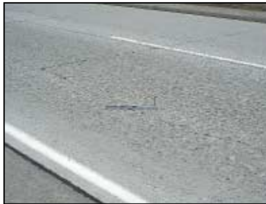
FIGURE 56 Distress Type JCP 3—Moderate Severity Longitudinal Cracking
