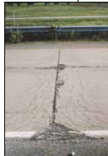
FIGURE 53 Distress Type JCP 2—High Severity “D” Cracking with Loose and Missing Material
