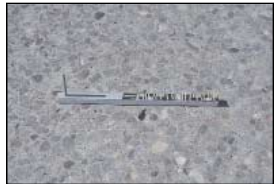
FIGURE 74 Distress Type JCP 10—A Popout
