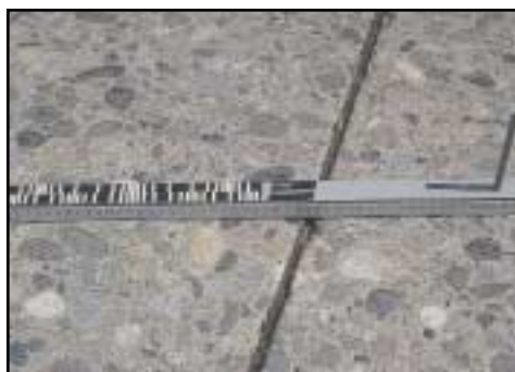
FIGURE 133 Distress Type CRCP 15—Longitudinal Joint Seal Damage
