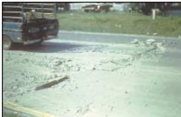
FIGURE 76 Distress Type JCP 11—A Blowup
