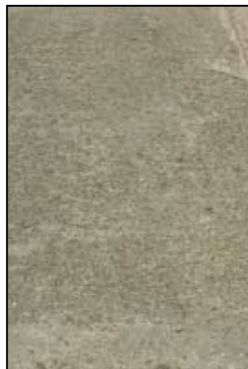
FIGURE 102 Distress Type CRCP 4b—Scaling
