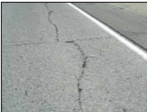
FIGURE 57 Distress Type JCP 3—High Severity Longitudinal Cracking
