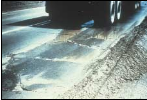
FIGURE 89 Distress Type JCP 16—Water Bleeding and Pumping
