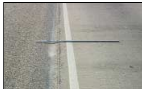
FIGURE 115 Distress Type CRCP 9—Lane-to-Shoulder Dropoff
