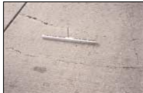
FIGURE 124 Distress Type CRCP 12—Low Severity Punchout
