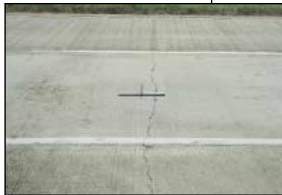
FIGURE 99 Distress Type CRCP 3—Moderate Severity Transverse Cracking
