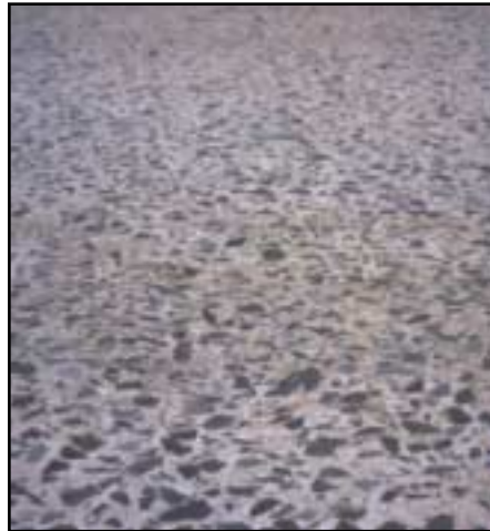
FIGURE 103 Distress Type CRCP 5—Polished Aggregate
