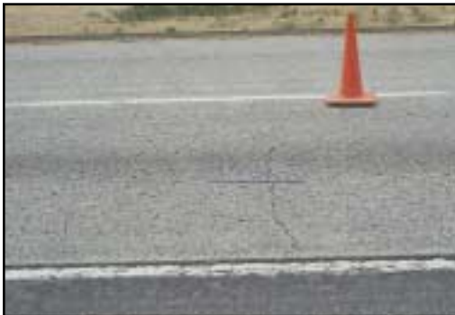
FIGURE 98 Distress Type CRCP 3—Low Severity Transverse Cracking
