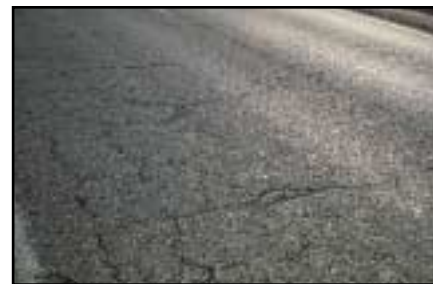
FIGURE 10 Distress Type ACP 2—High Severity Block Cracking
