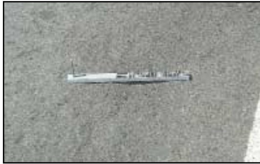
FIGURE 40 Distress Type ACP 13—Loss of Fine Aggregate
