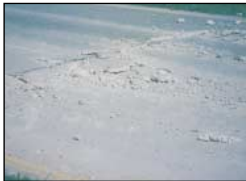
FIGURE 107 Distress Type CRCP 7—A Blowup
