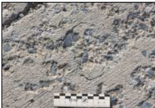
FIGURE 71 Distress Type JCP 8b—Scaling, Close-up View
