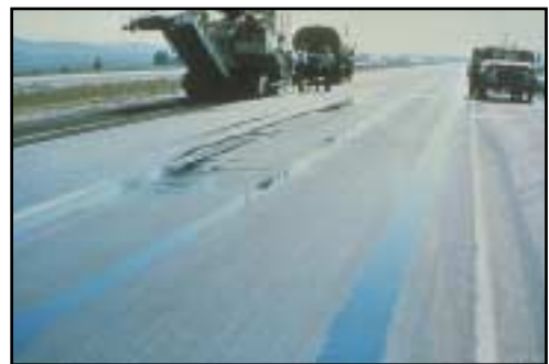
FIGURE 33 Distress Type ACP 9—Standing Water in Ruts
