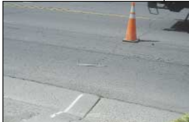
FIGURE 20 Distress Type ACP 6—Moderate Severity Transverse Cracking
