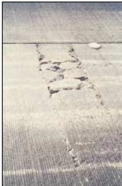
FIGURE 126 Distress Type CRCP 12—High Severity Punchouts
