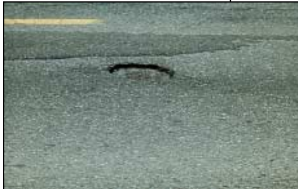
FIGURE 28 Distress Type ACP 8—Moderate Severity Pothole
