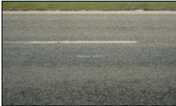
FIGURE 36 Distress Type ACP 11—Discoloration
