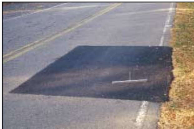
FIGURE 24 Distress Type ACP 7—Low Severity Patch
