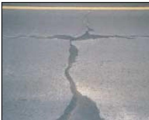
FIGURE 45 Distress Type ACP 15—Water Bleeding and Pumping
