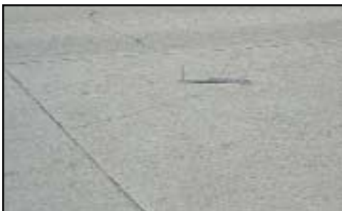
FIGURE 49 Distress Type JCP 1—Low Severity Corner Break
