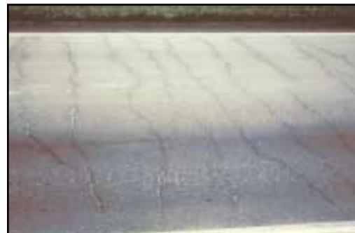
FIGURE 97 Distress Type CRCP 3—Transverse Cracking Pattern
