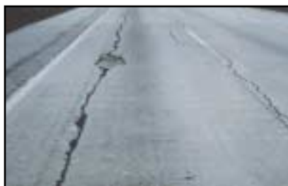
FIGURE 95 Distress Type CRCP 2—High Severity Longitudinal Cracking
