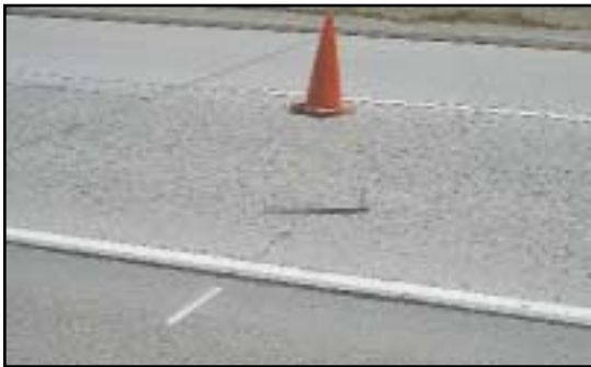
FIGURE 59 Distress Type JCP 4—Moderate Severity Transverse Cracking
