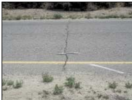
FIGURE 21 Distress Type ACP 6—High Severity Transverse Cracking
