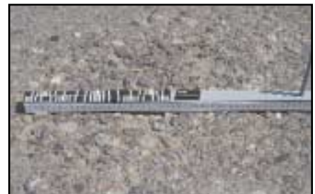
FIGURE 42 Distress Type ACP 13—Loss of Coarse Aggregate
