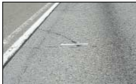
FIGURE 50 Distress Type JCP 1—Moderate Severity Corner Break
