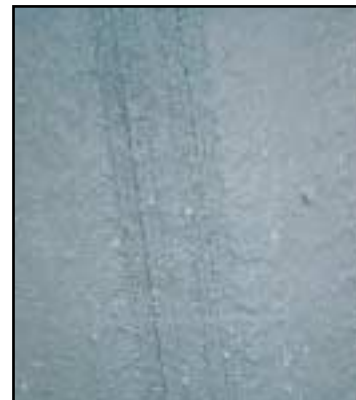
FIGURE 38 Distress Type ACP 11— Aggregate Obscured
